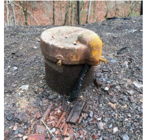
Burned well head after a wildfire. Photo used by permission from the Tennessee Department of Health.
