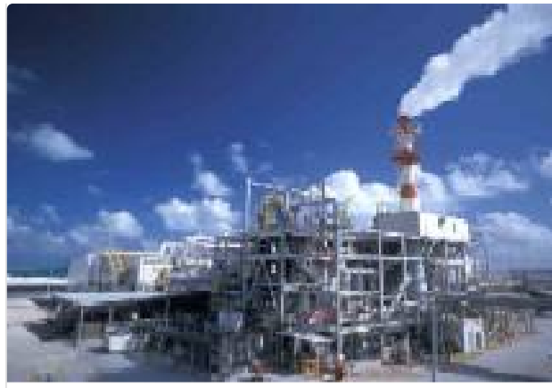
Chemical Weapons Elimination Facility, Johnston Atoll
