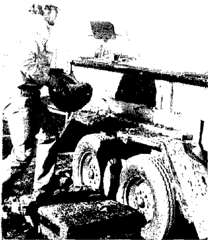
FIGURE 2. Worker getting ready to "drop" asphalt into a roofing kettle.
