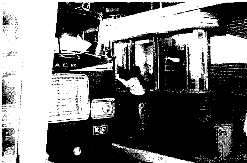
FIGURE 3. Toll collection booth and plaza canopy.
