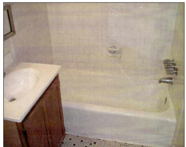
Photo courtesy of Maryland Occupational Safety and Health
