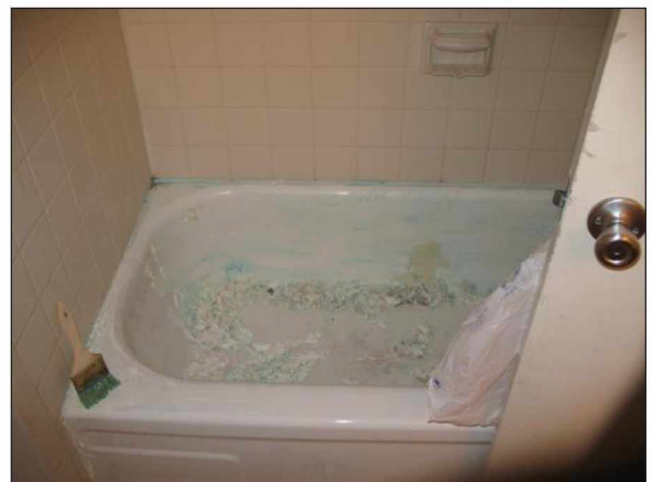
A bathtub painted with a stripping chemical used during the reglazing process.
