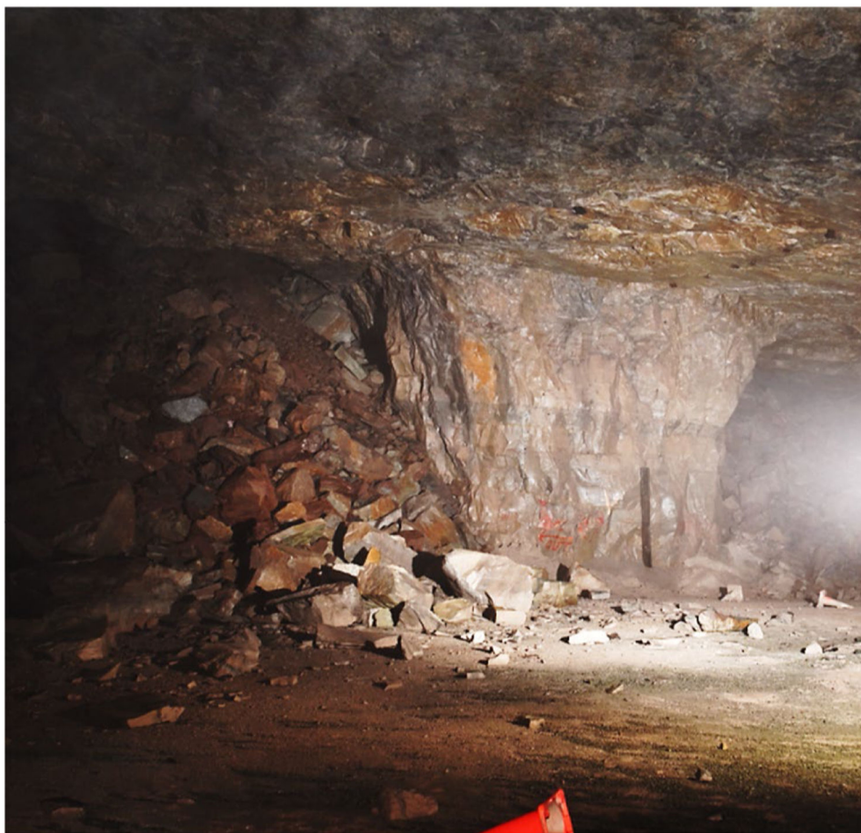
Fig. 8. Rubble from the roof collapse and a stable pillar along the edge of the area that collapsed
