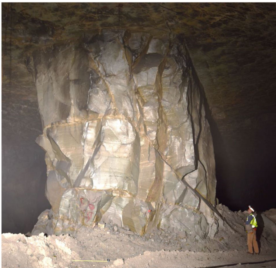
Fig. 4. Prominent N60°W striking joint intersecting a pillar south of the collapsed area
