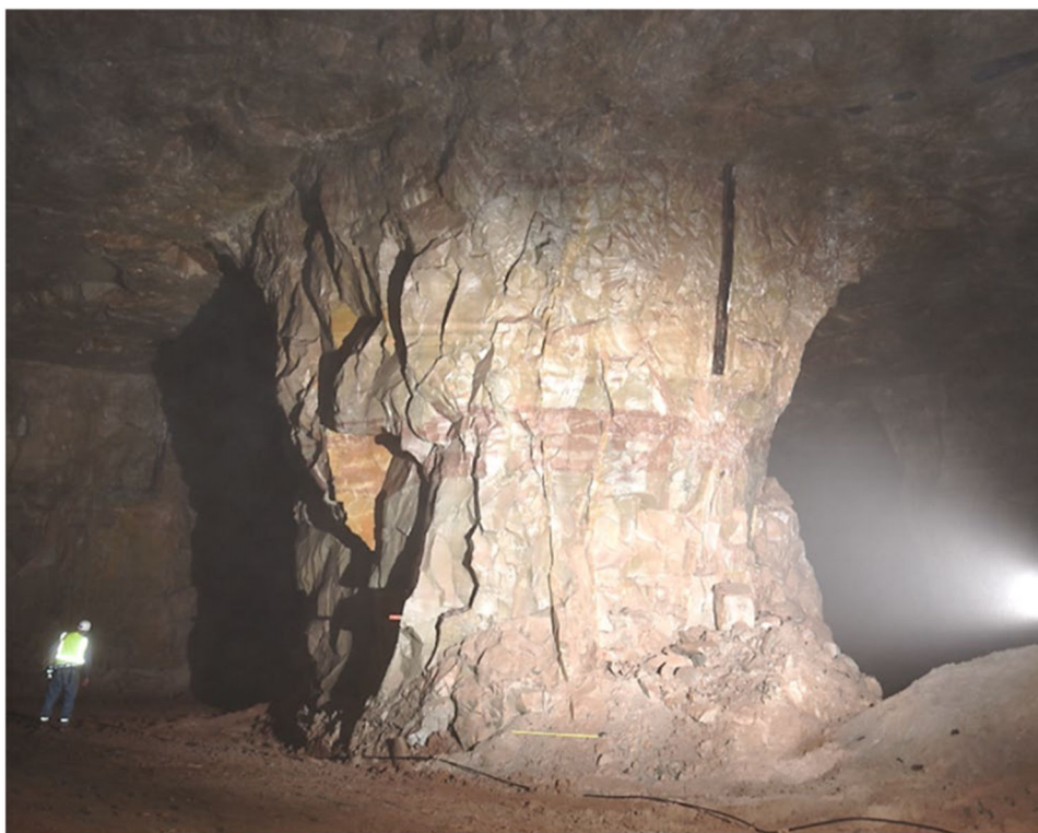
Fig. 7. Pillar affected by angular jointing adjacent to the collapsed area
