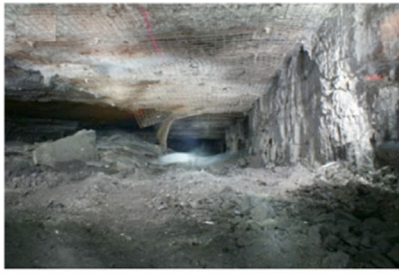
(a) Bearing capacity failure
