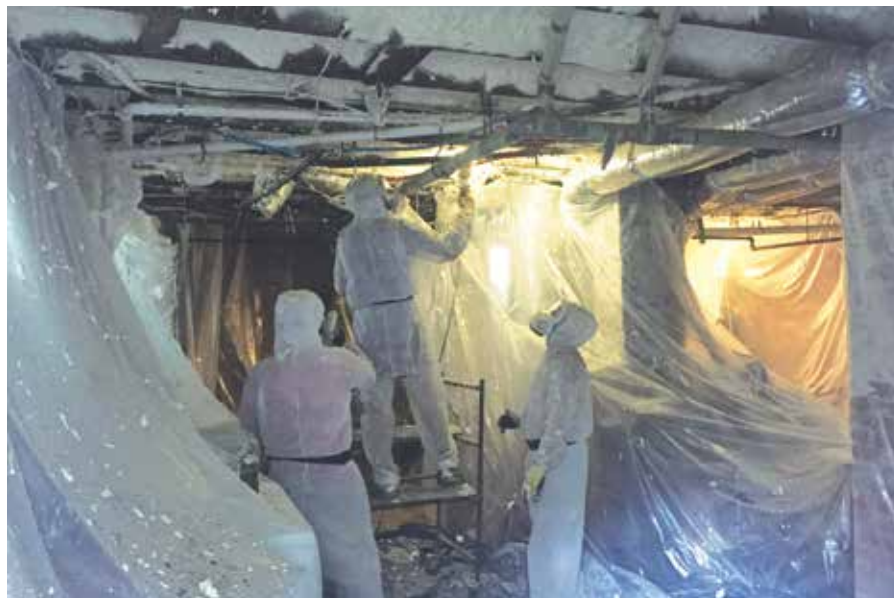
Application of spray polyurethane foam insulation in the basement an existing home.
