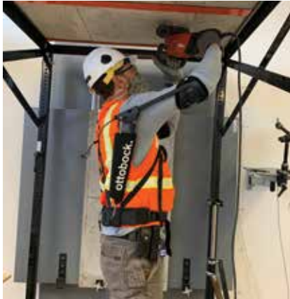
Researchers grind concrete overhead, a common but physically challenging activity, while supported with an exoskeleton.
