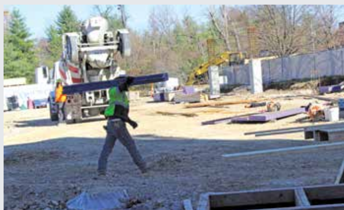
Manual materials handling on a St. Louis-area job site.
