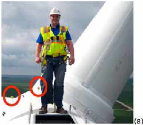
Figure 1. (a) 5,000 lb Anchorage Points for Tie Off (b) Factory Installed Ladder System with Fall Arrest (from Bowen Engineering)
