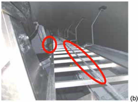
Figure 1. (a) 5,000 lb Anchorage Points for Tie Off (b) Factory Installed Ladder System with Fall Arrest (from Bowen Engineering)
