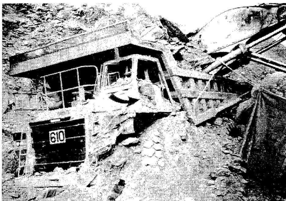
Truck buried in highwall failure that resulted in one fatality and one nonfatal injury
