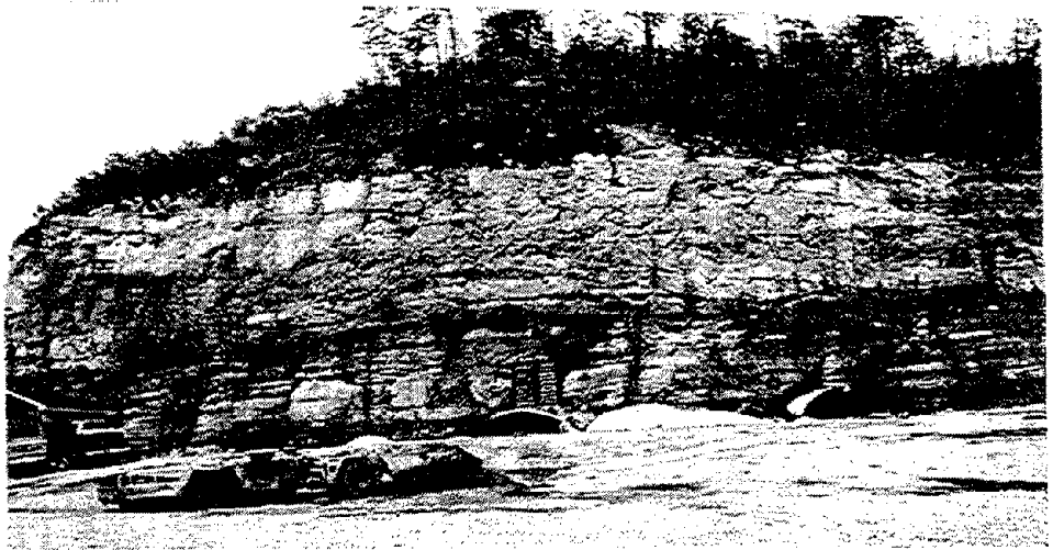
A near-vertical highwall at an Appalachian drift coal mine that poses a serious hazard to workers
