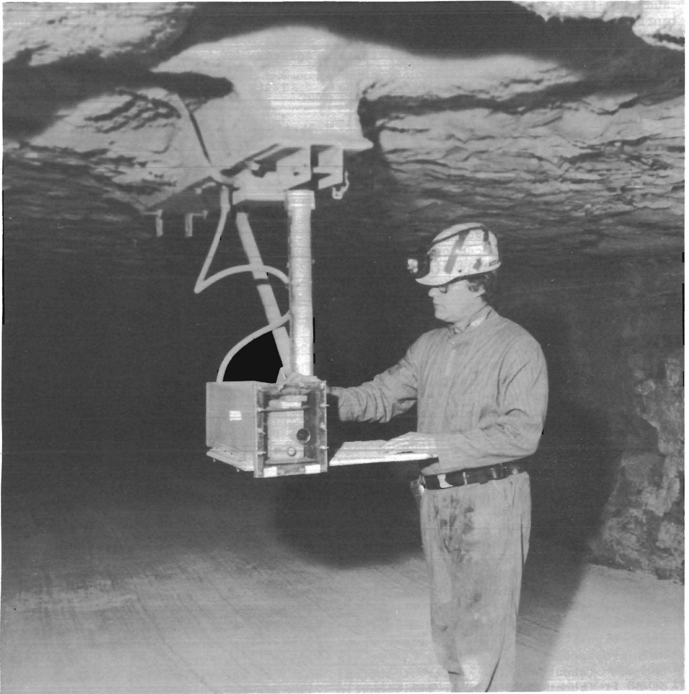
FIGURE 5.—Retractable sensor platform with high-speed camera in D-drift.
