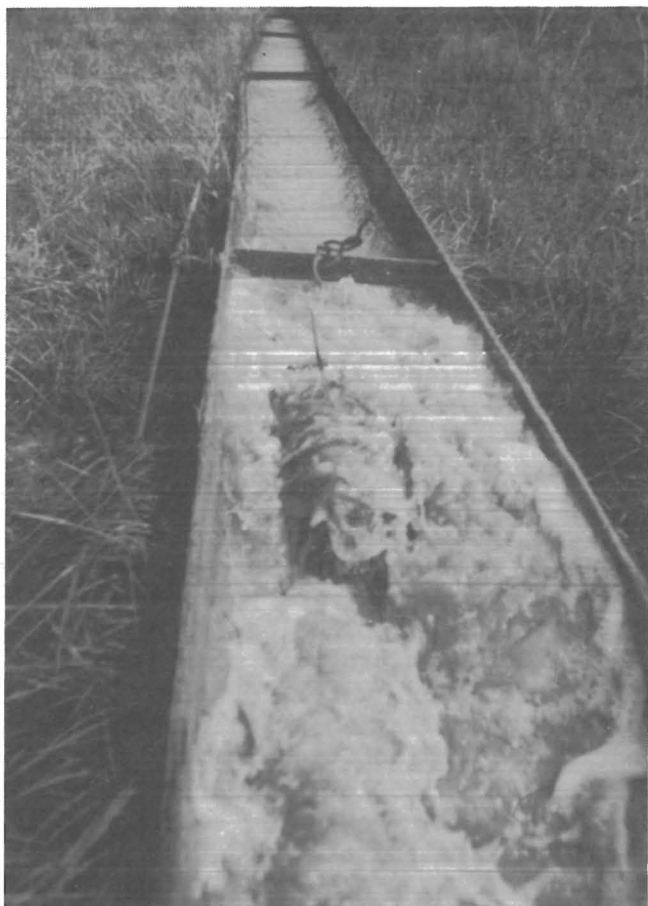
FIGURE 12. - Gel log installation in flume.
