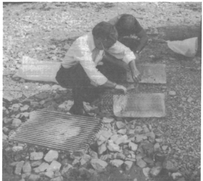
FIGURE 11. • Gel logs being wrapped in chicken wire.
