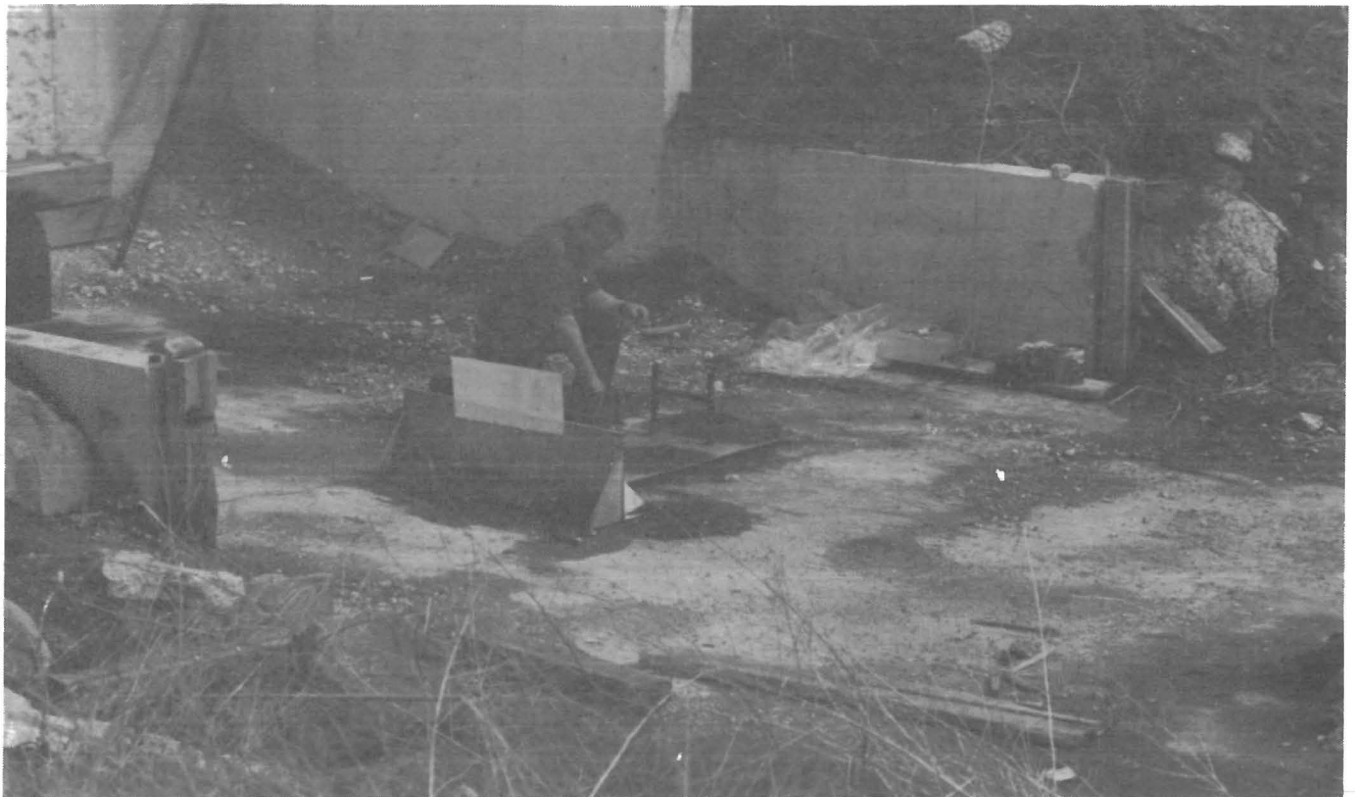
FIGURE 7. - Setting velocity-measurement trip wires.
