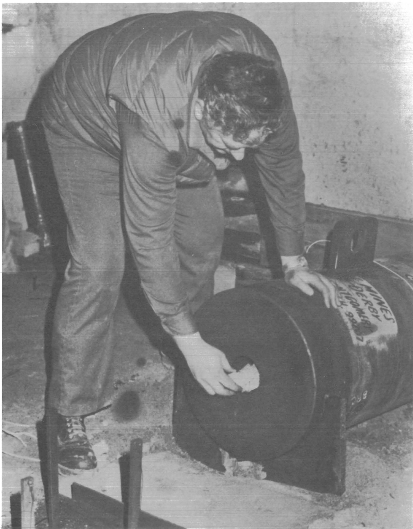
FIGURE 8. - Installing primer cord charge.
