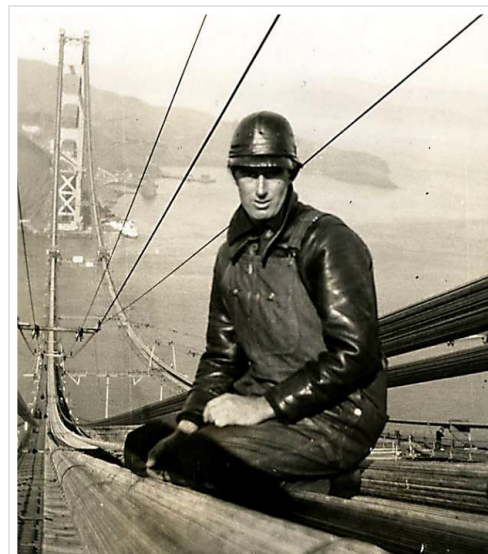
A Golden Gate construction worker wears a Bullard “hard boiled hat” in this photograph, circa 1936. Credit: Labor Archives and Research Center, J. Paul Leonard Library, San Francisco State University.
