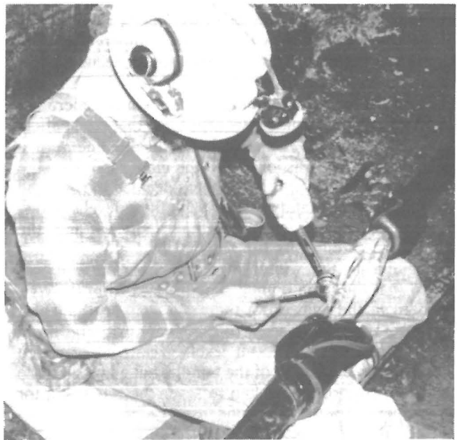
Figure 5.—Splicing main tube bundle during installation of pneumatic fire detection system.
