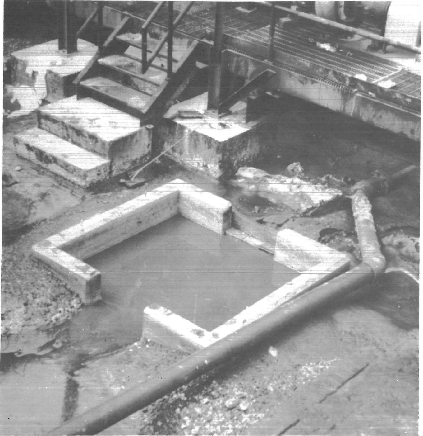
FIGURE 10.—Sulfur concrete sump unit in industrial corrosive environment.
