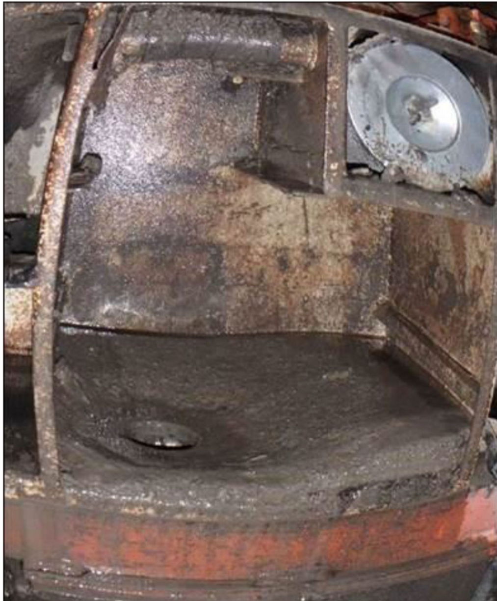
Fig. 2. Dry dust collector box that has been converted to the wet box.
