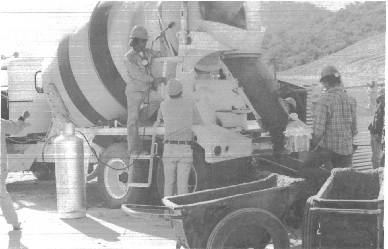
FIGURE 7. - Modified ready-mix truck used in production of sulfur concrete.
