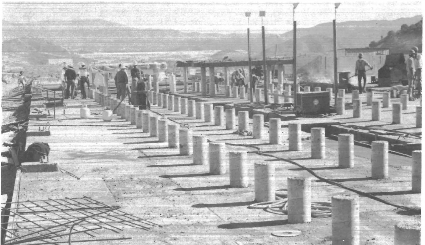
FIGURE 13. - Finished sulfur concrete floor.
