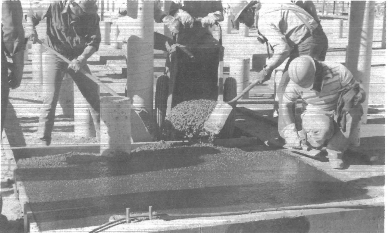
FIGURE 12. - Installing sulfur concrete floor in an electrolytic copper plant.
