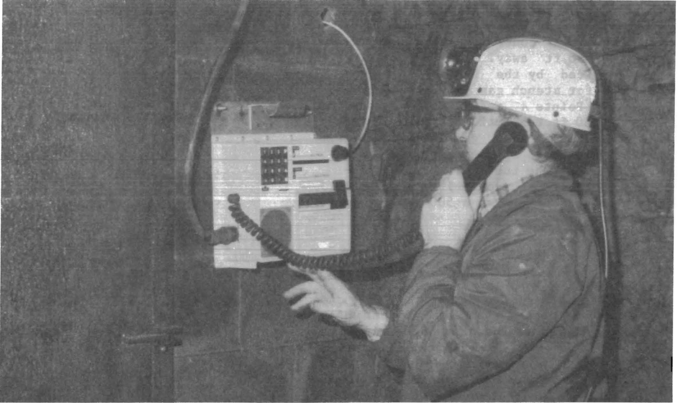
FIGURE 3. • Receiver phone mounted on outside of intake shaft at mine level.
