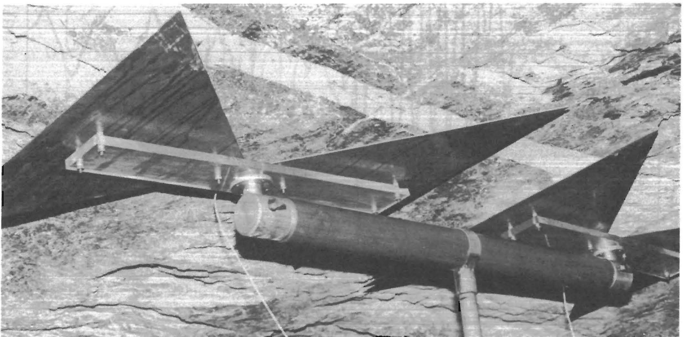
FIGURE 6. - Antenna installation against mine roof.
