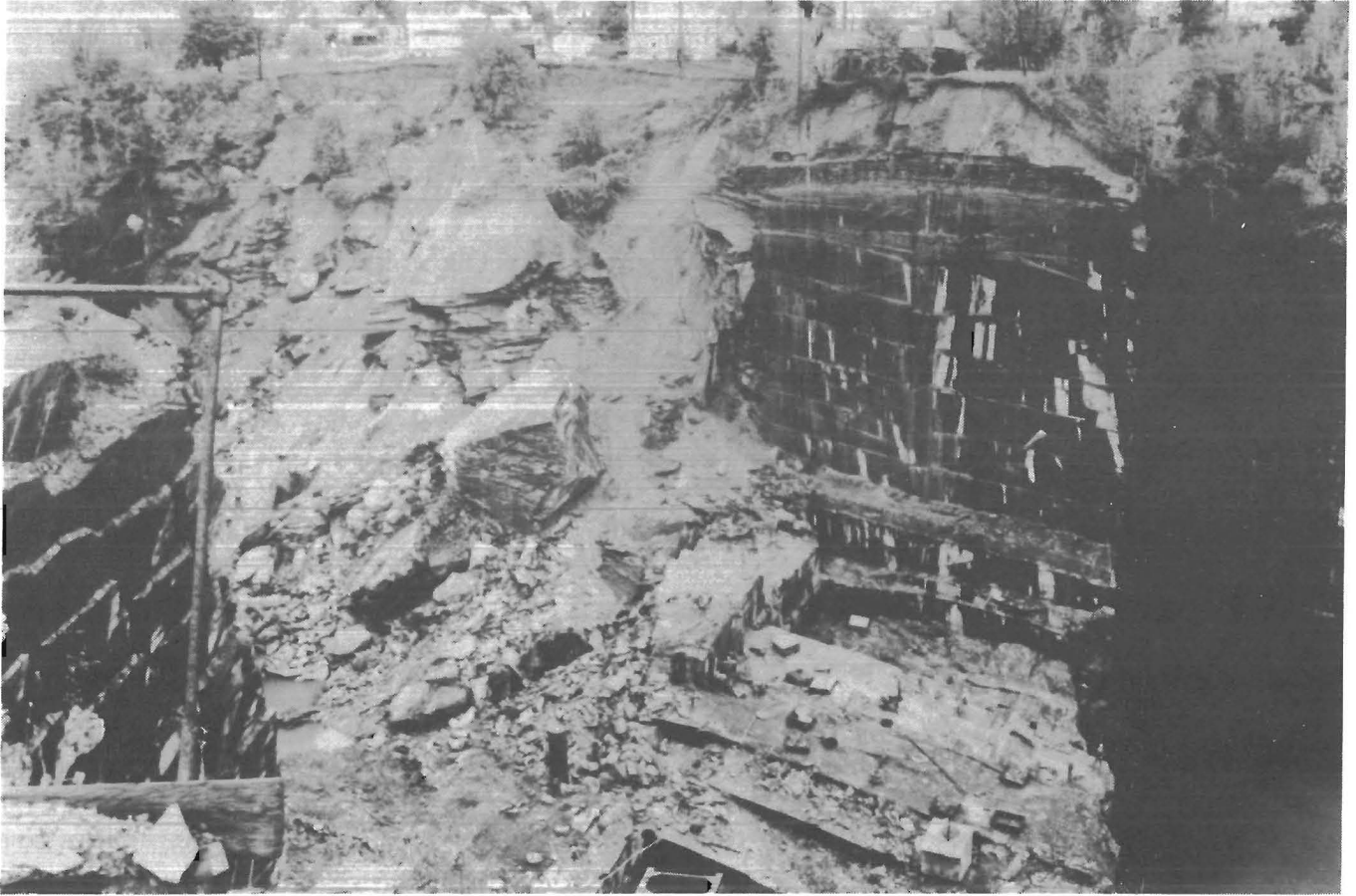
FIGURE 15. - Collapse of quarry highwall adjacent to operating section.
