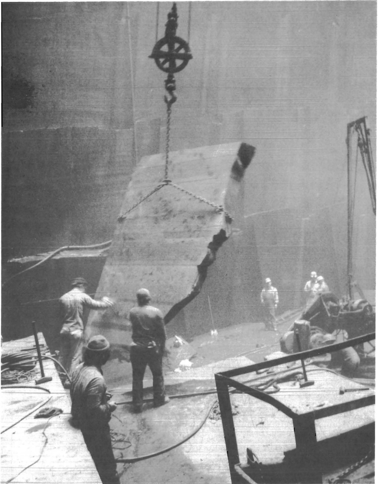
FIGURE 3. - Method of hoisting slate slabs to surface.
