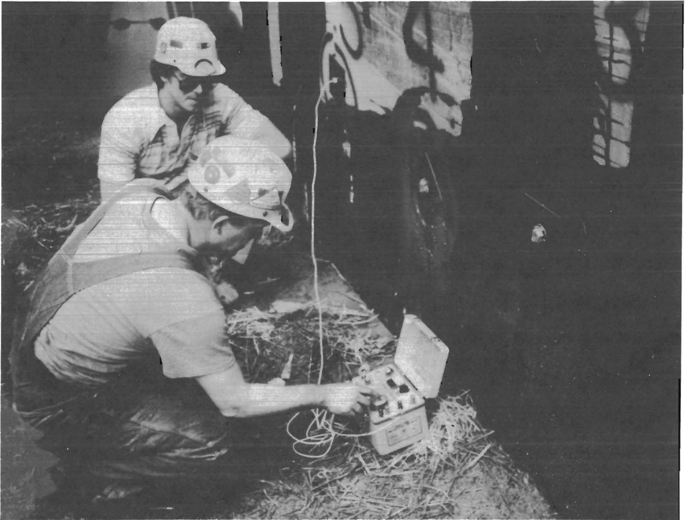
FIGURE 34. - Measuring rockbolt tension bleedoff.
