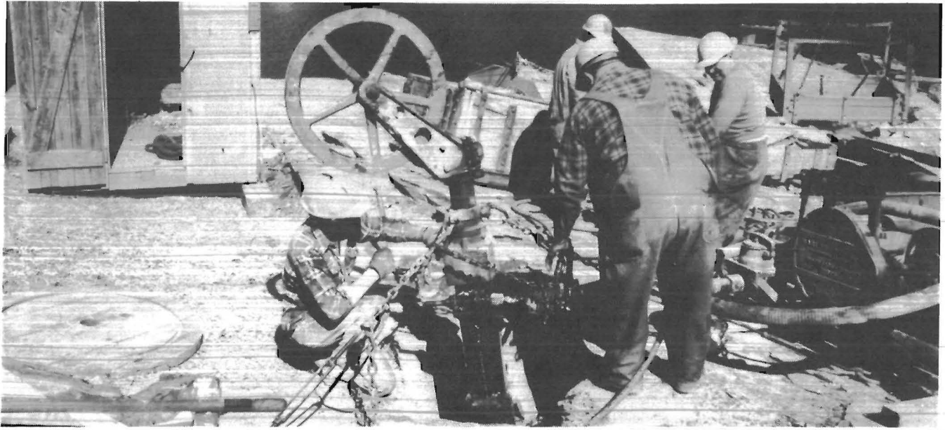
FIGURE 4. - Installing standard and sheave for wire rock-sawing operation.
