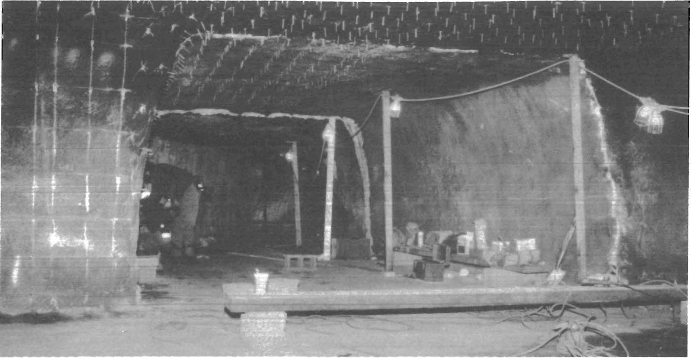
Figure 3.—Installation of fireproof material at test site.
