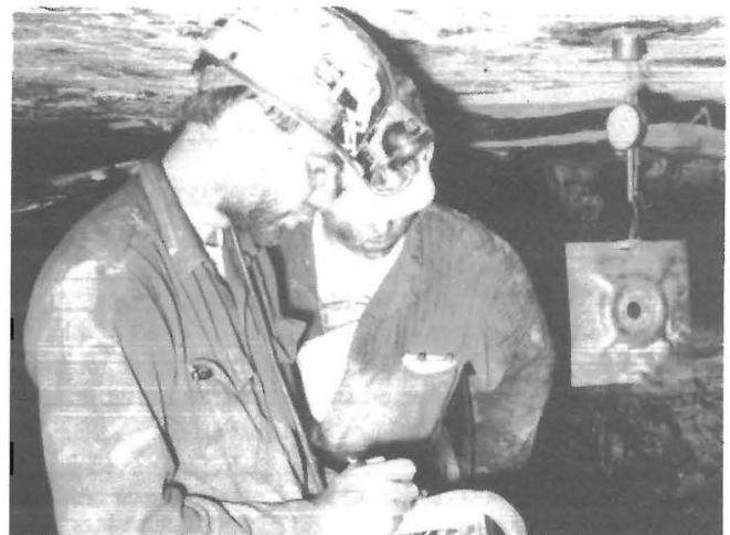
Figure 6.-Bureau engineers measuring roof sag.
