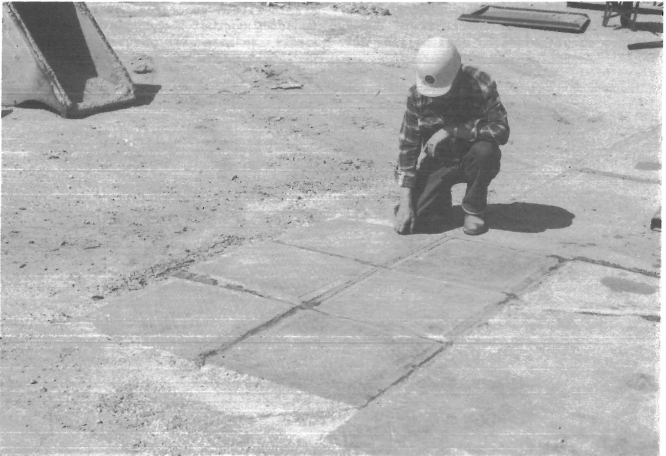
FIGURE 6. - Fiber concrete slabs installed in front of laboratory building.
