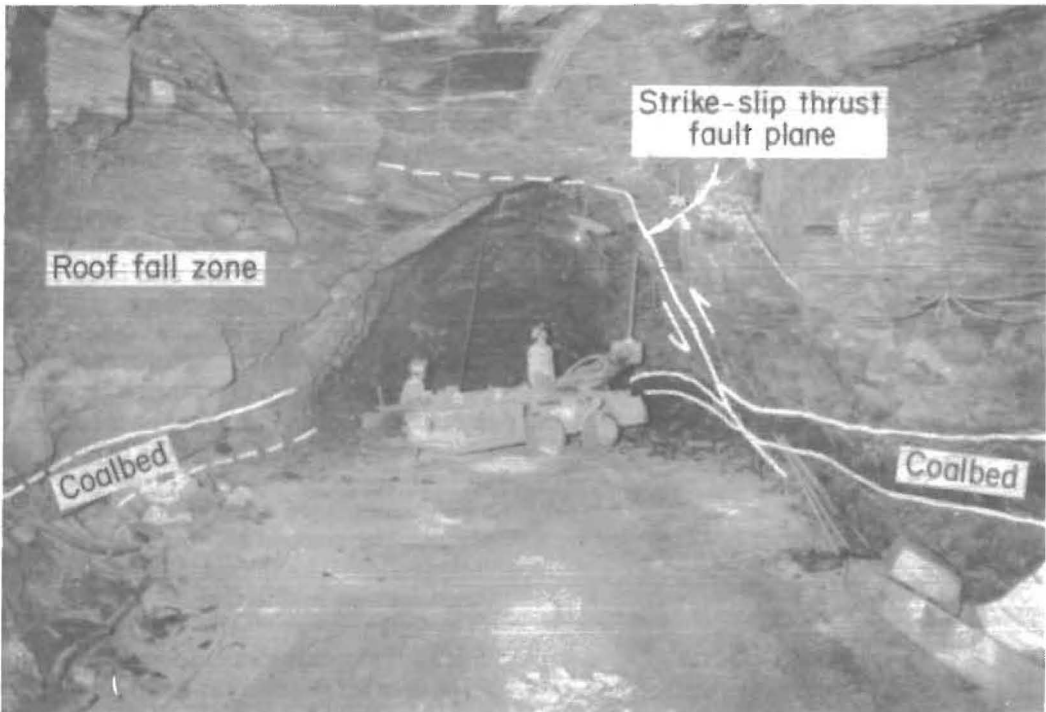
Figure 10.-Rehabilitation of high-roof fall in entry crossing Pistol Gap Fault zone.
