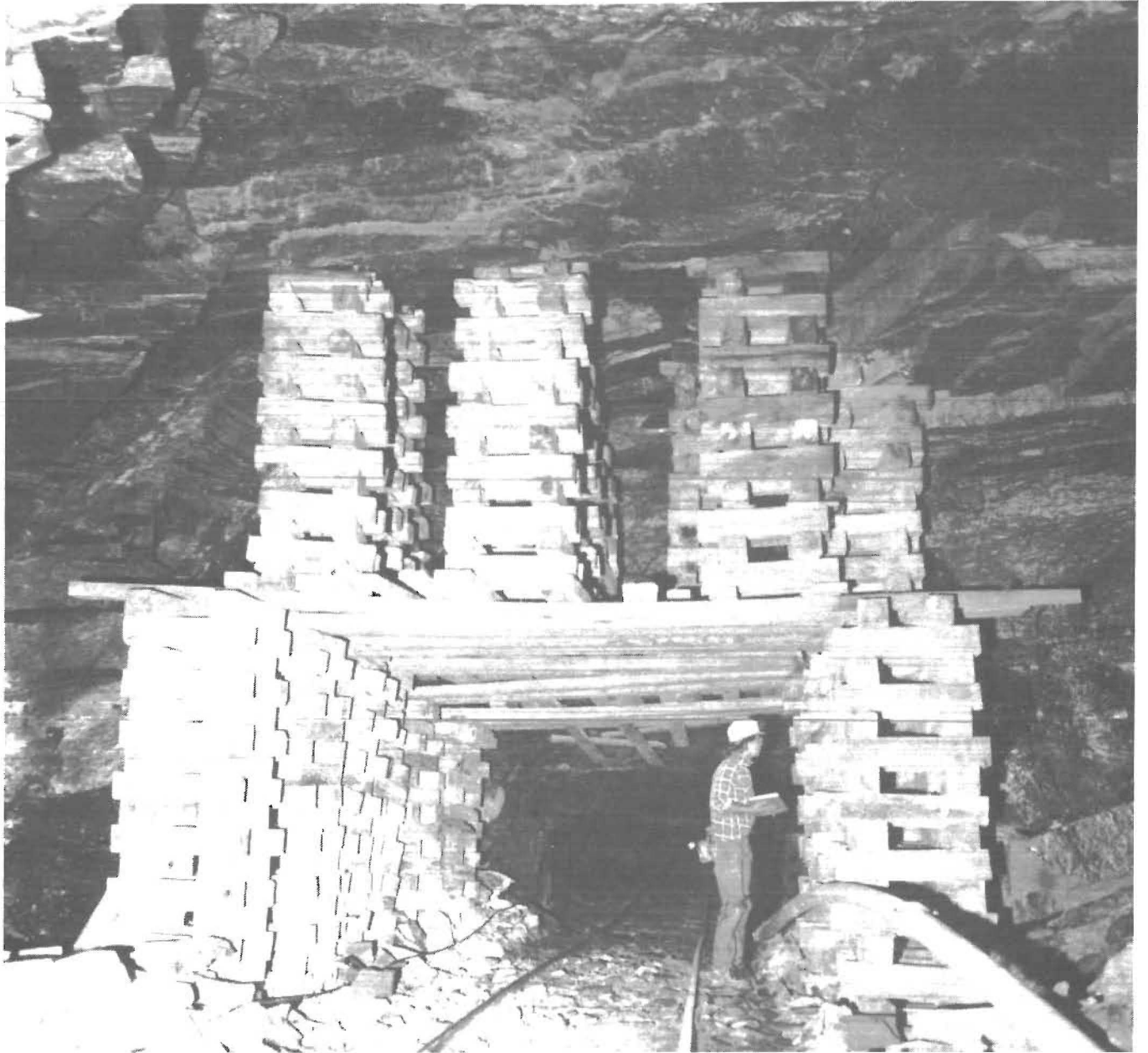
Figure 15.-Two-tiered cribbing platform, built to support high-roof fall in Chaparal Mine.
