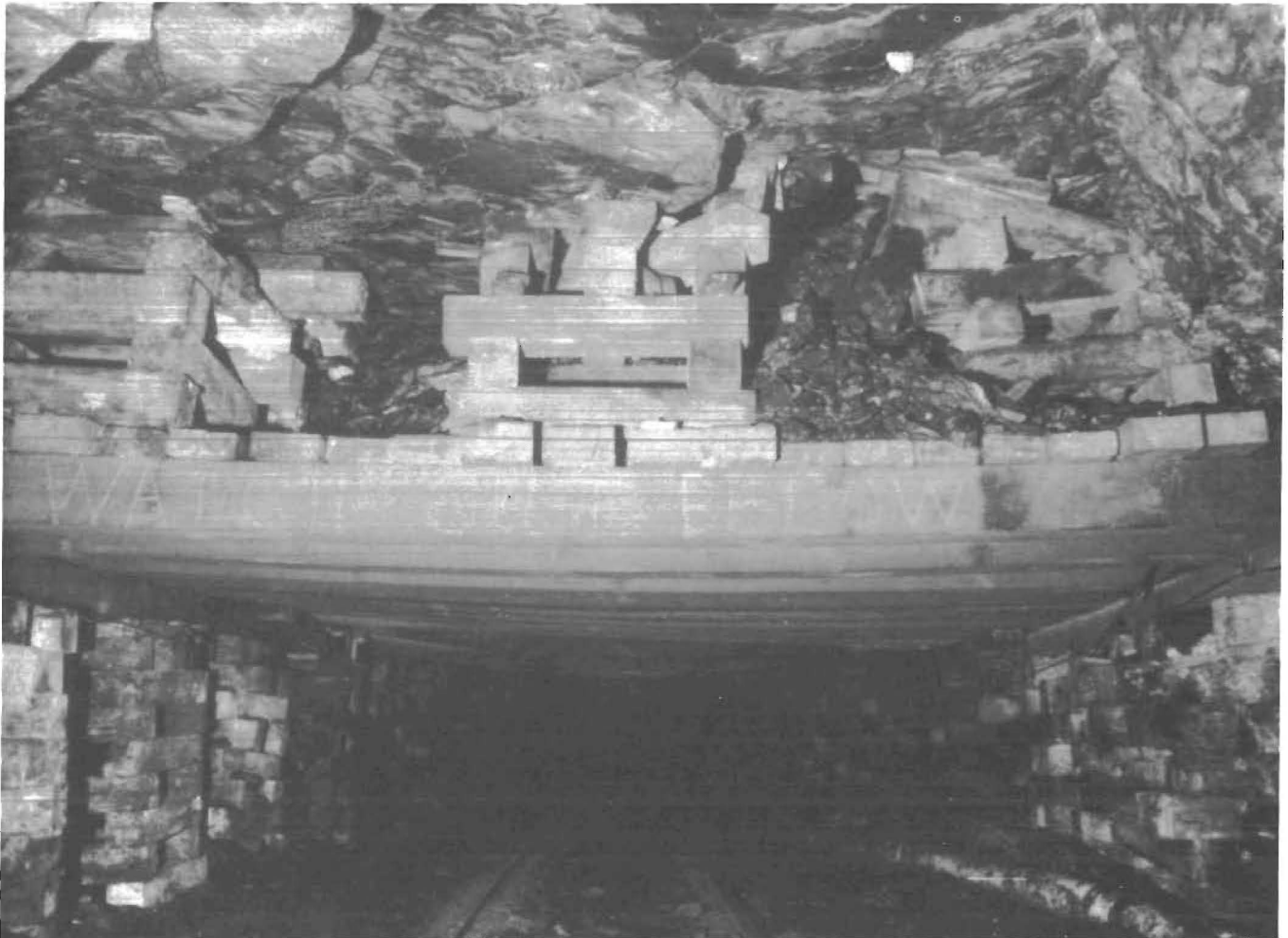
Figure 27.—Permanent structure used to support roof through fault zone.
