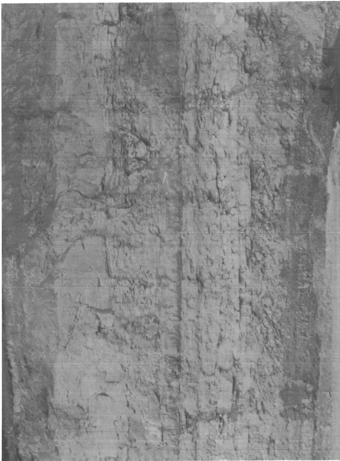
FIGURE 8. - Right stereomodel, test wall, 250-ms delays in the highwall holes.
