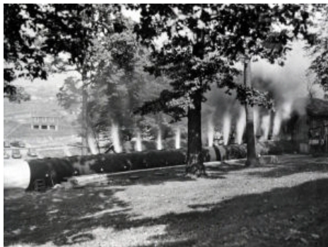
Gallery for testing explosives
