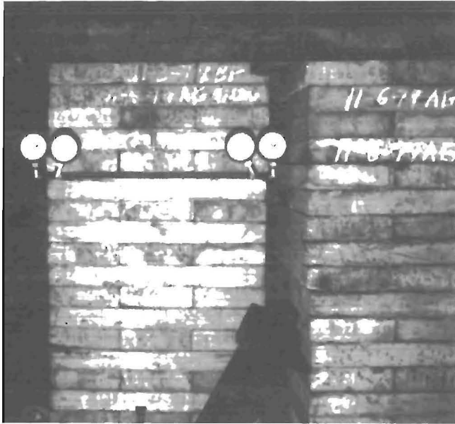
FIGURE 4. - Panel 10 left instrumentation layer installed in first SFC crib.
