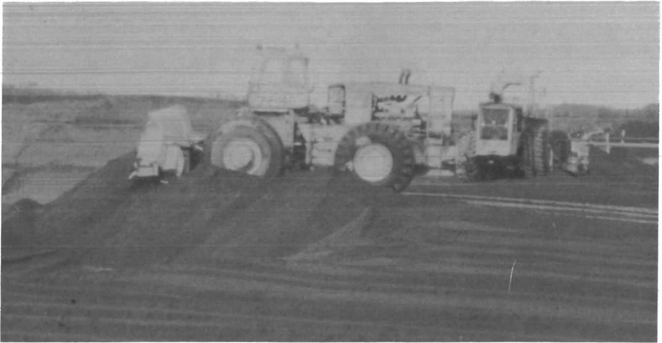
FIGURE 9. - Embankment crest being built.
