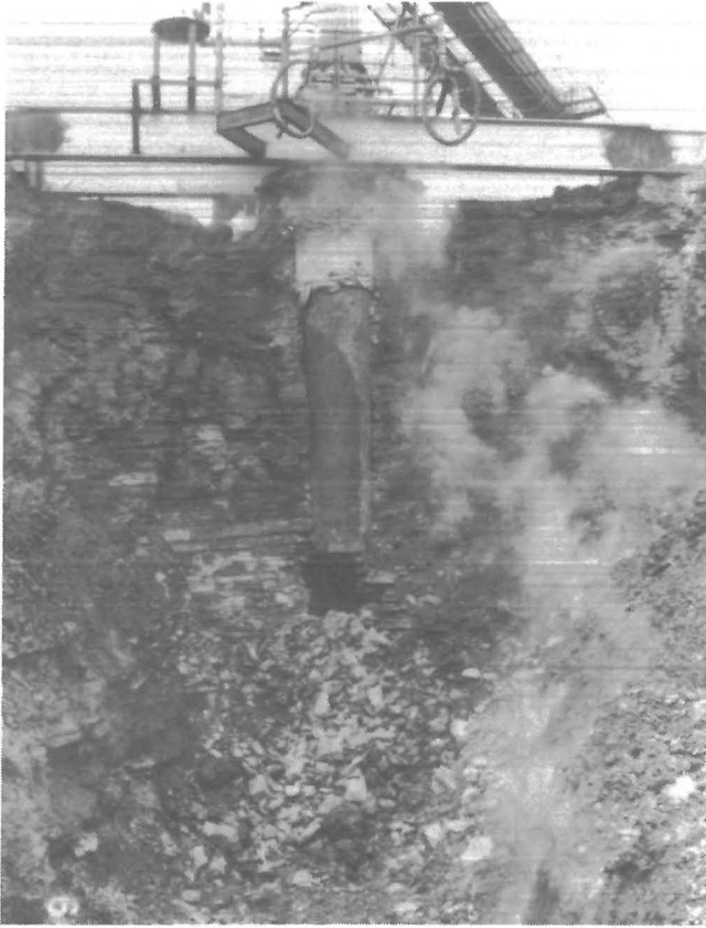
FIGURE 10. - Exposed exhaust manifold.
