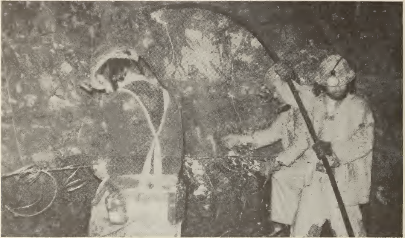
FIGURE A-10. - Loading explosives into blast holes in the face of a drift.
