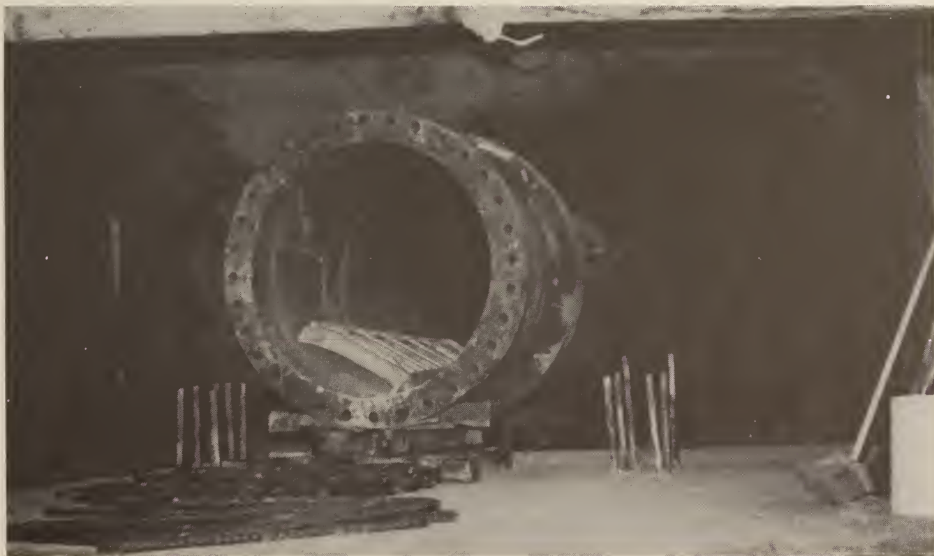
FIGURE A-15. - Ventilation duct being installed underground.
