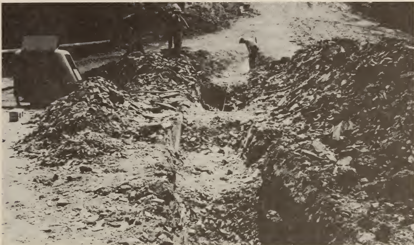
FIGURE A-4. - Cutting utility trench in solid rock near the fanhouse.
