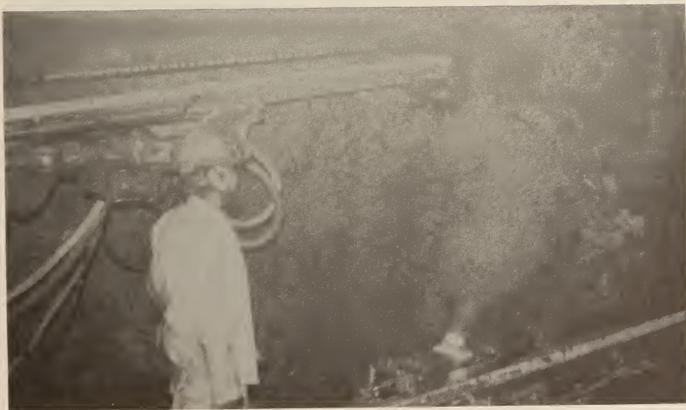
FIGURE A-9. - Drilling in preparation for a blast in drift driving.
