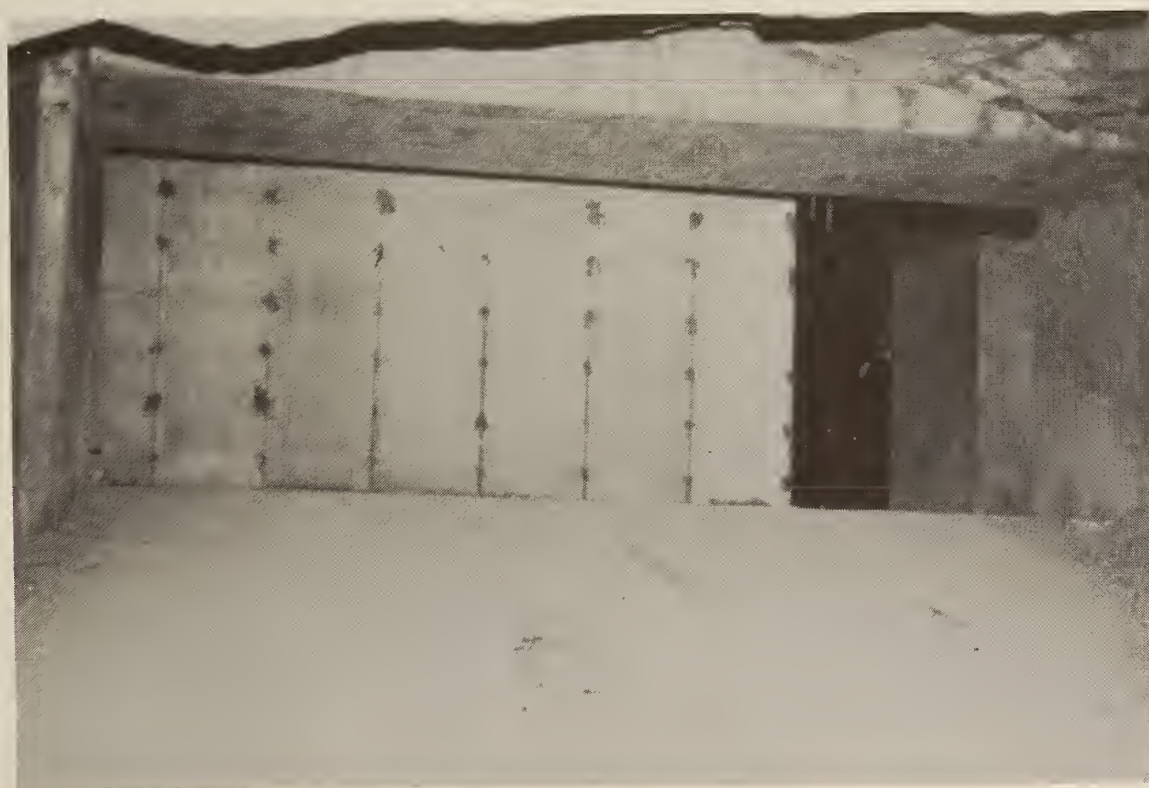
FIGURE 13. - Movable bulkhead in partially closed position.
