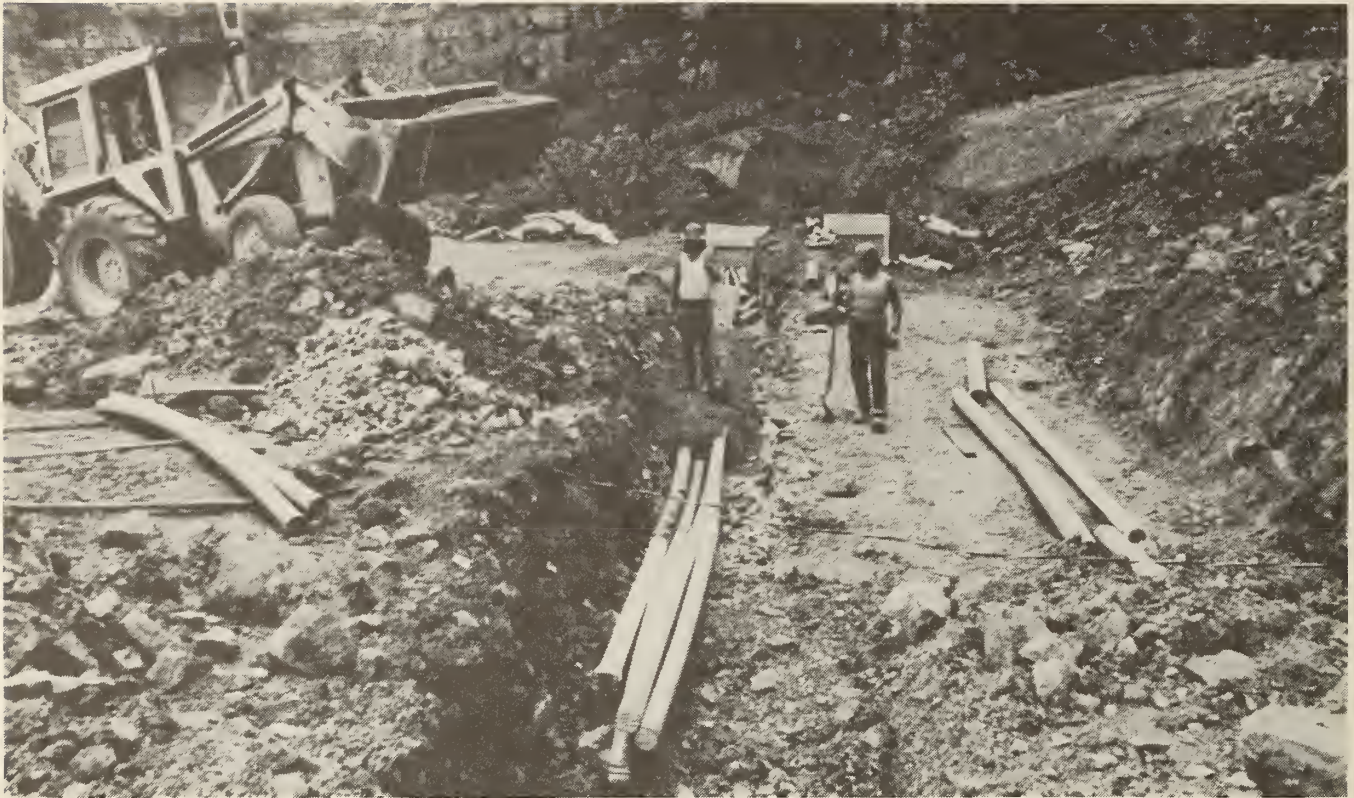
FIGURE A-6. - Installing conduits in solid limestone paralleling the highwall between the control building and the underground workings.
