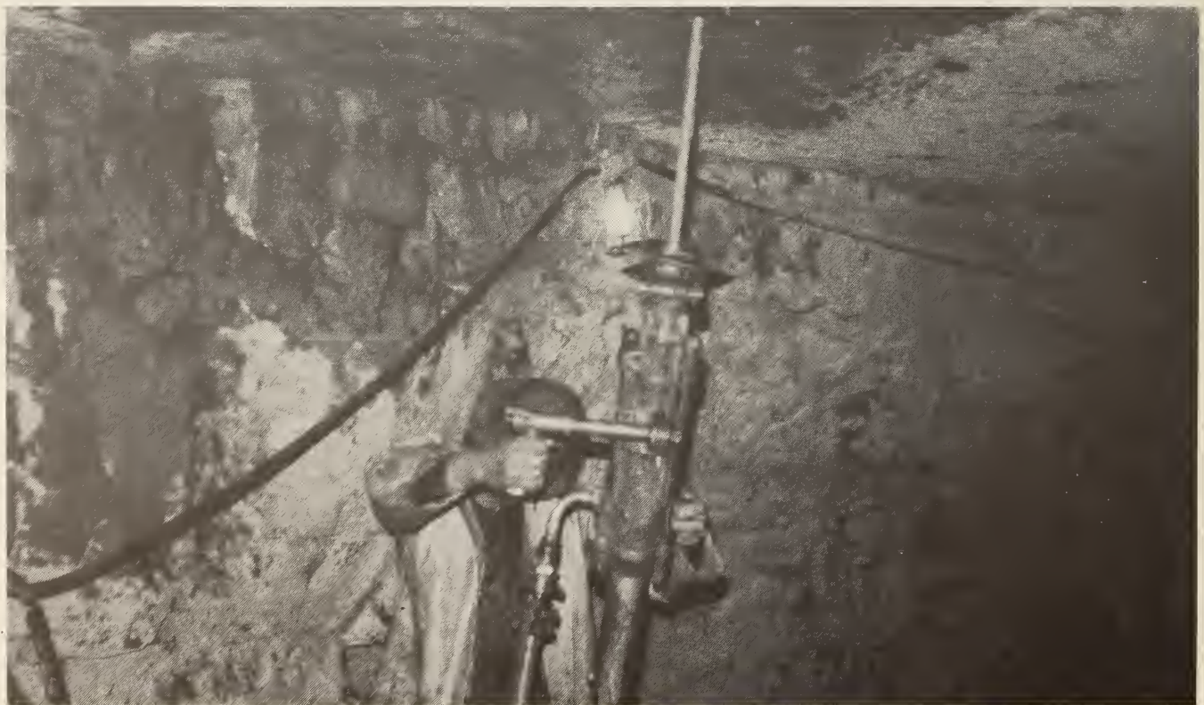
FIGURE A-17. - Installation of 4-ft roof bolt in a drift.
