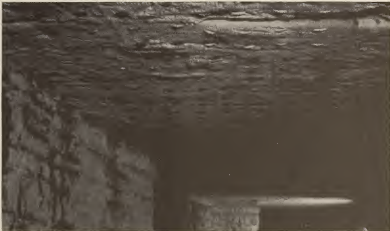
FIGURE A-18. - Roof bolt pattern in the old workings in areas being used as transporting routes.
