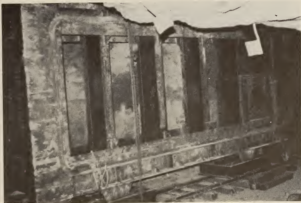
FIGURE 12. - Movable bulkhead before installation of reinforcing rods and pouring of concrete.
