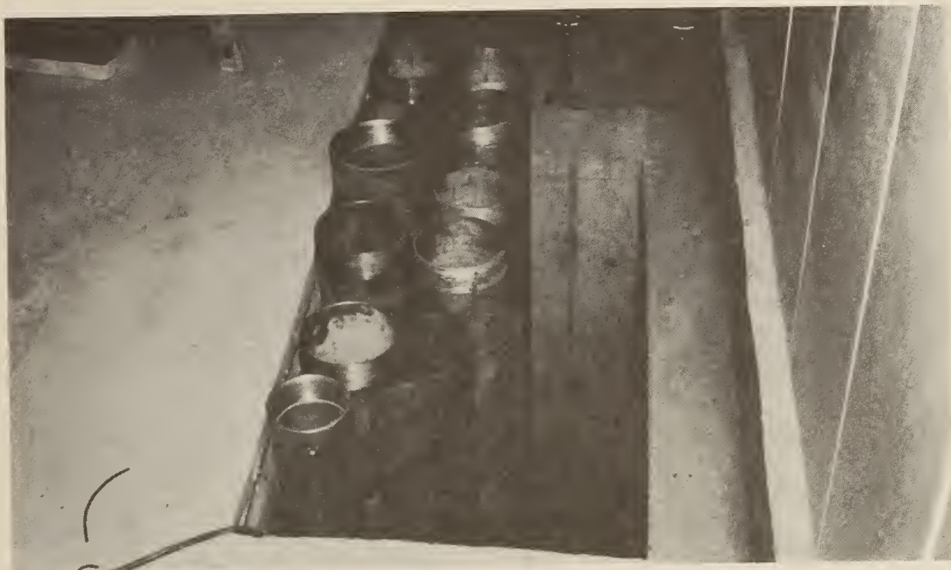
FIGURE A-8. - Conduits from underground entering computer room.
