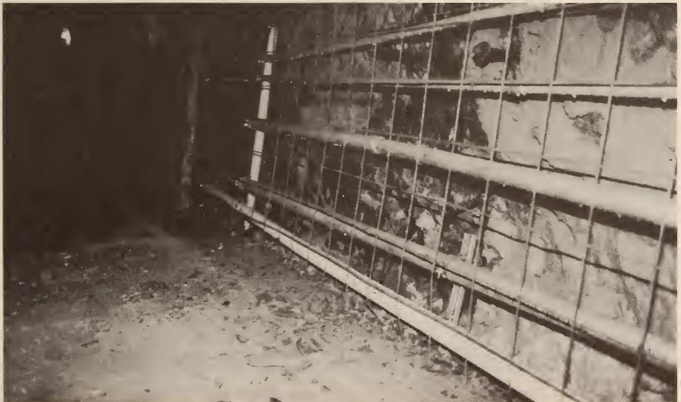
FIGURE 34. - Forming and reinforcement for the concrete fenders underground; these fenders encase the air and water lines and the power, communication, and instrument cables.
