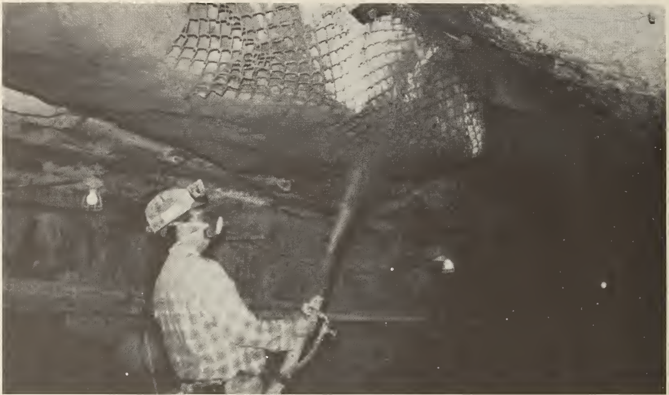
FIGURE A-16. - Installing gunite (fibrous) on a fault in B-drift.
