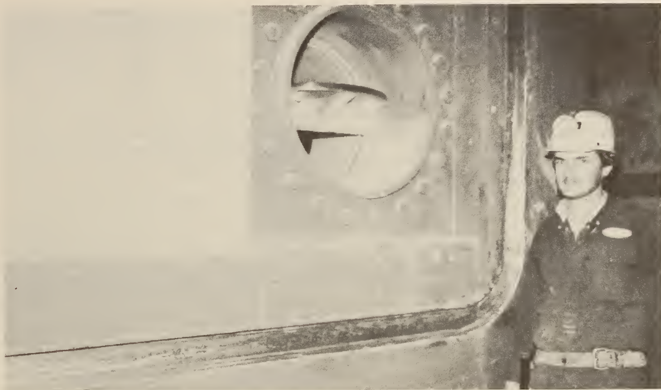
FIGURE 16. - Remote-controlled 24-in butterfly valve installed in movable bulkhead.
