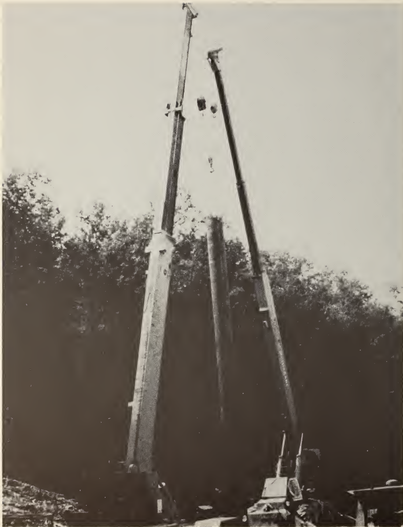
FIGURE A-13. - Two cranes lowering a 2-ft casing into a vertical borehole.
