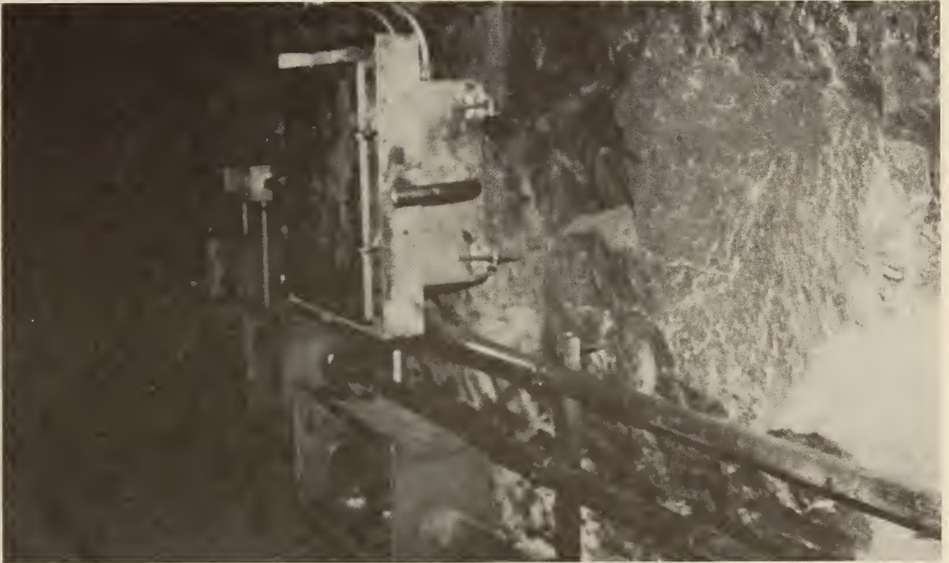
FIGURE 33. - DG panel—before pouring of concrete fender.
