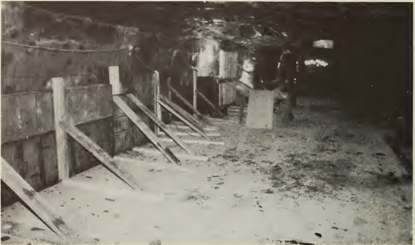
FIGURE A-20. - Forms to hold wet concrete for fender to protect instrumentation and utility, power, air, and water lines.
