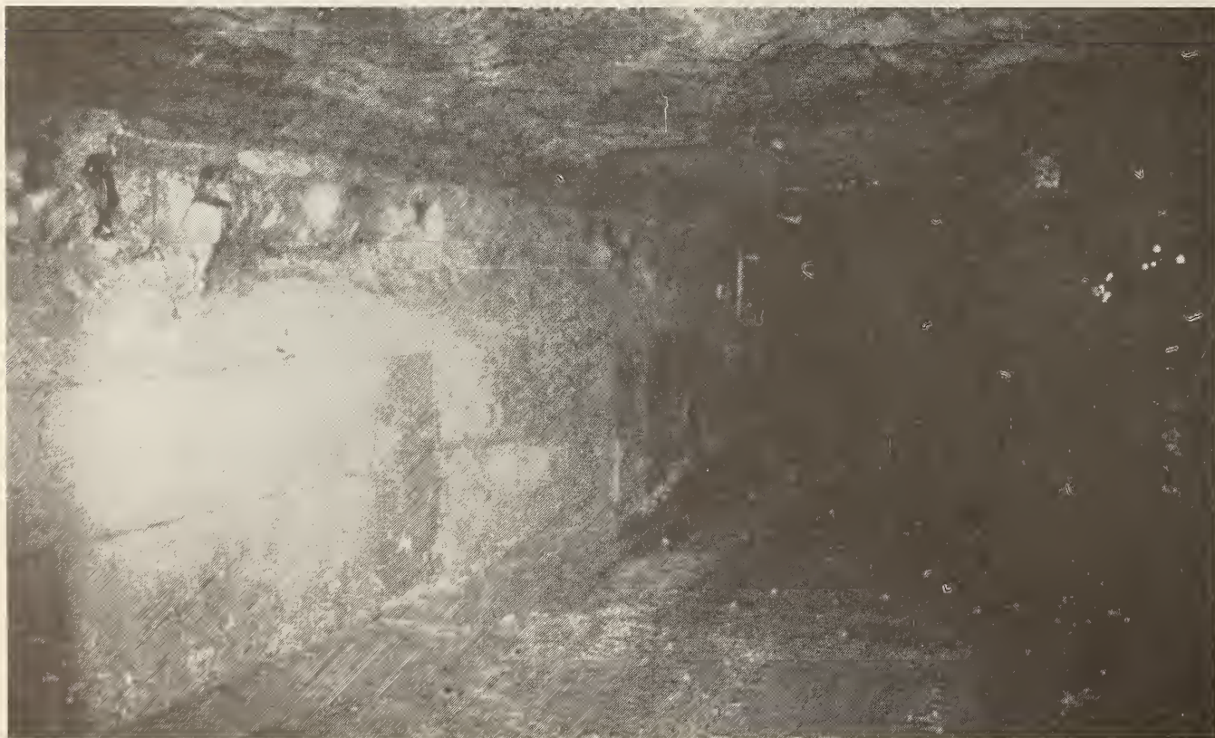
FIGURE 35. - View of a completed drift showing concrete floor and rib with concrete fender.
