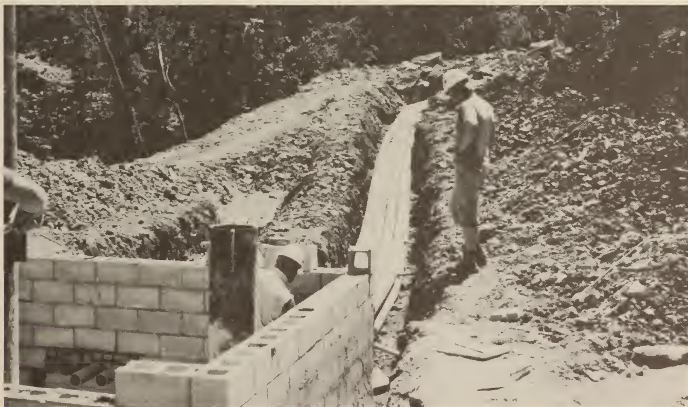
FIGURE A-5. - Installing conduits from one utility pit to another.
