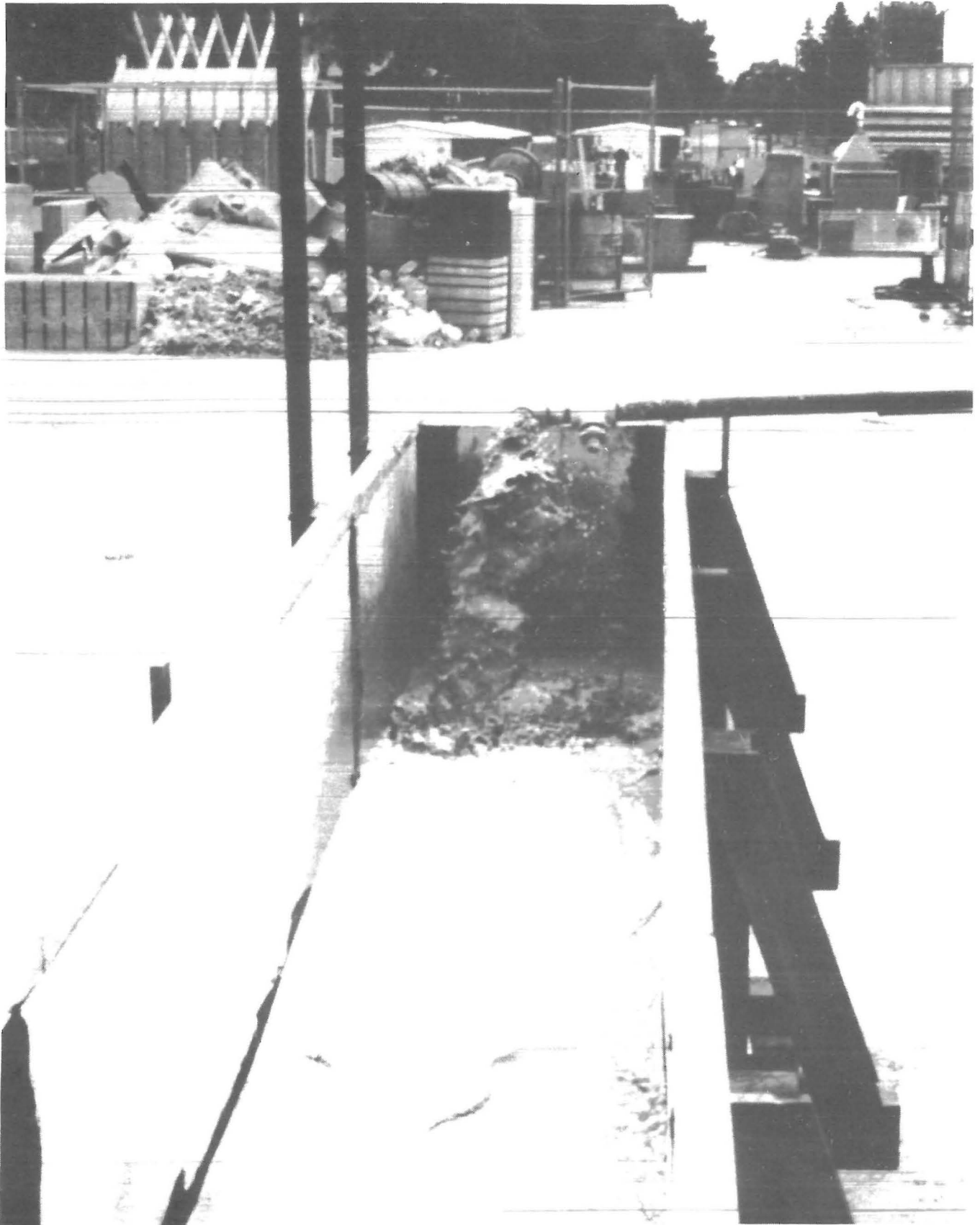
FIGURE 6.--Depositing tailings to form beach in trough.
