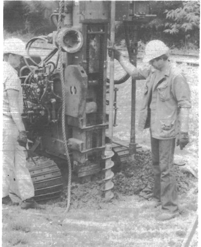
Figure 5.—Split spoon being lowered into hollow-stem auger hole.
