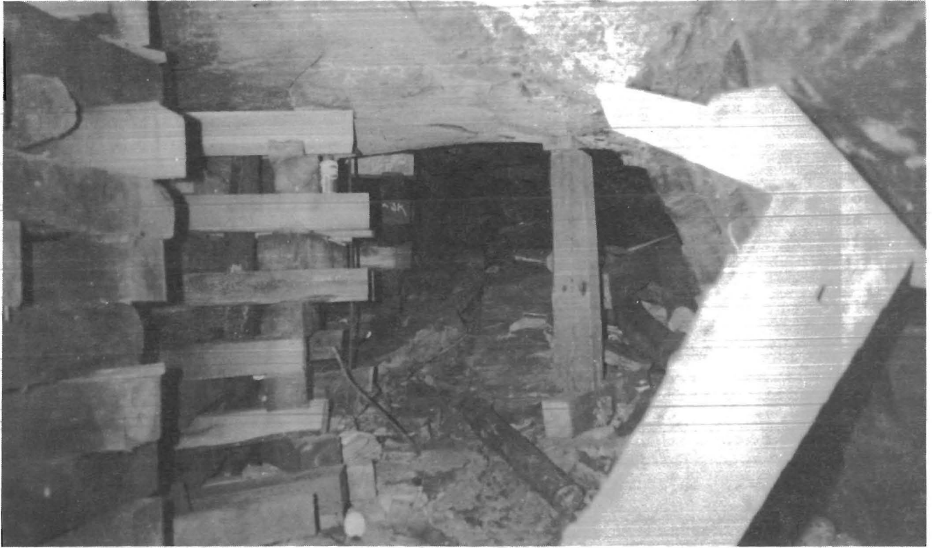
FIGURE 2.—Cribbing and posts used as temporary supports.
