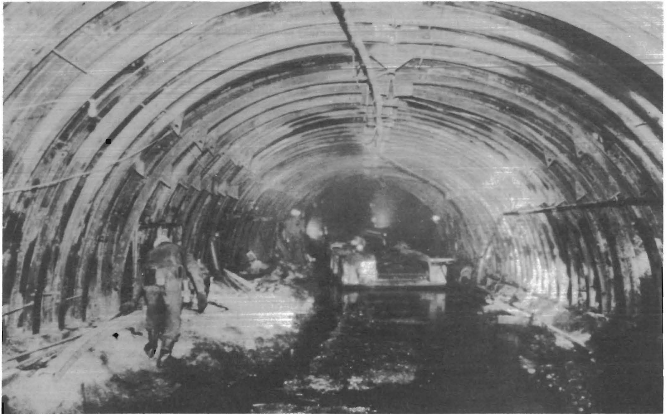
FIGURE 14.—Liner plate arch with inner arch supports. (Courtesy Camber Corp.)
