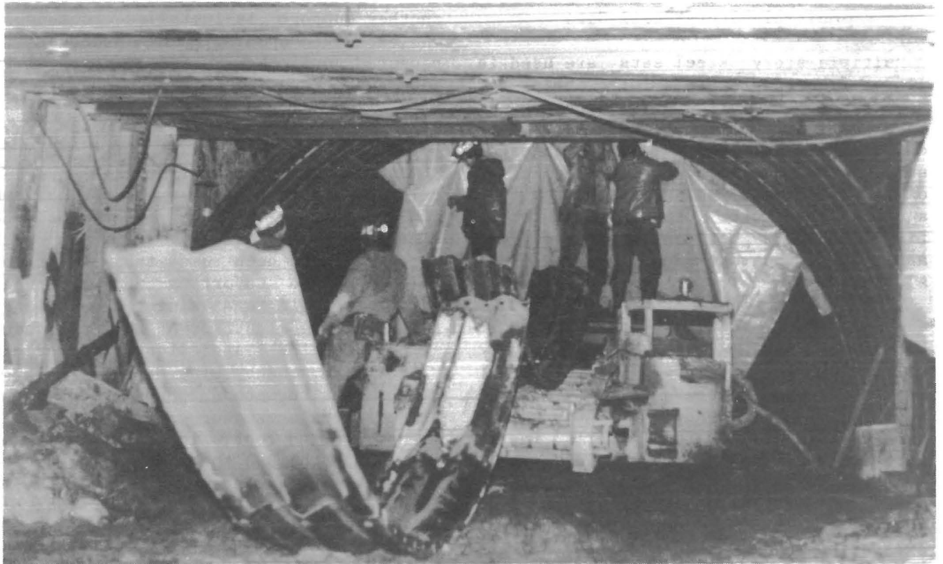
FIGURE 10.—Erection of liner plate arch. (Courtesy Camber Corp.)
