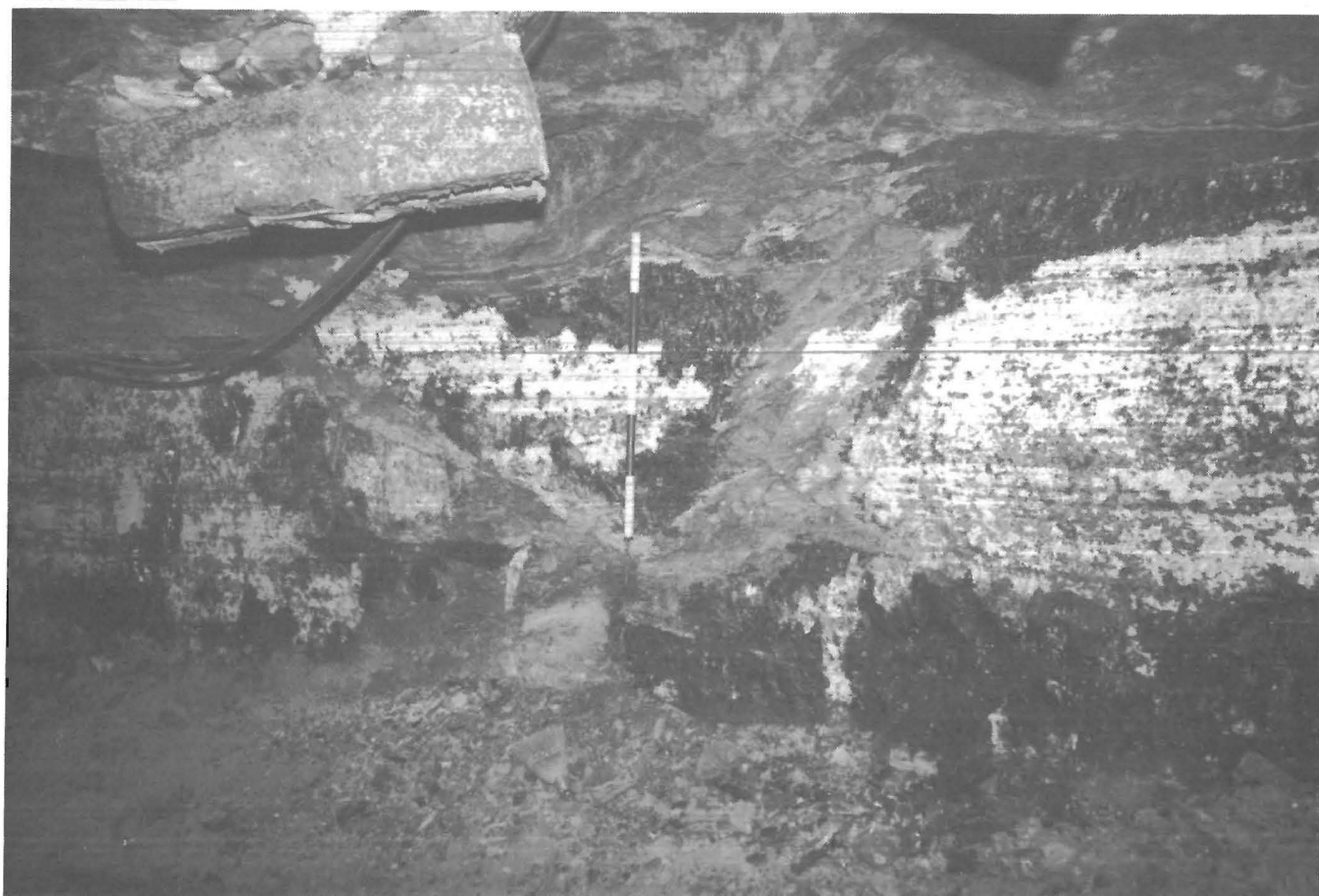
FIGURE 7.—Example of a clastic dike in both the mine roof and coal seam. (Courtesy F. E. Chase, BuMines, Pittsburgh, PA.)
