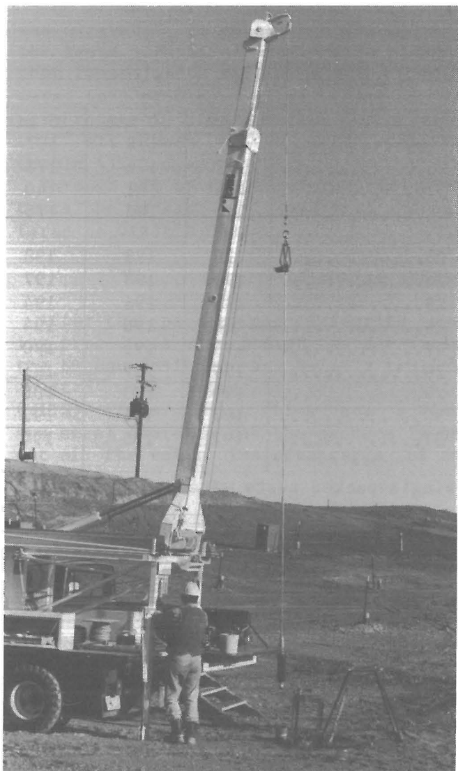
FIGURE 6. - Hoist truck lowering packer into well.
