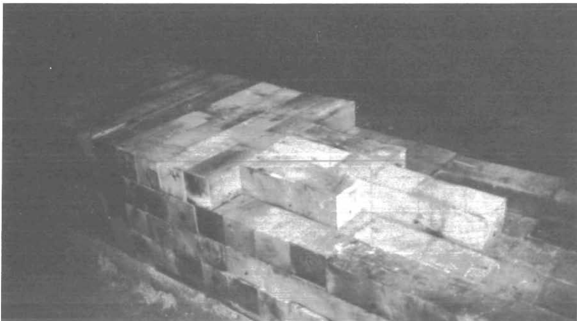
Figure 16.—Staggered wood-block joints.
