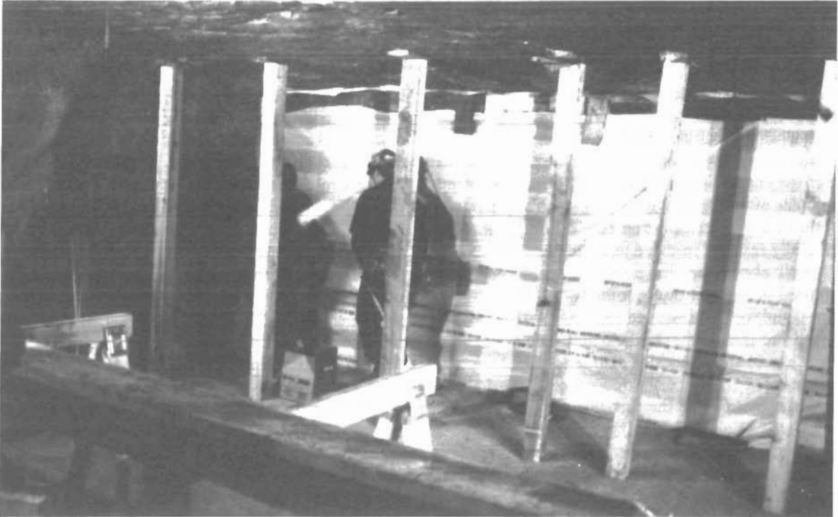
Figure 8.—Wooden framework for cementitious foam seal.
