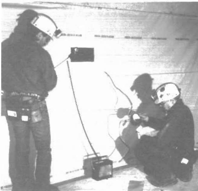
Figure 6.—Monitoring of air flow through test seal.
