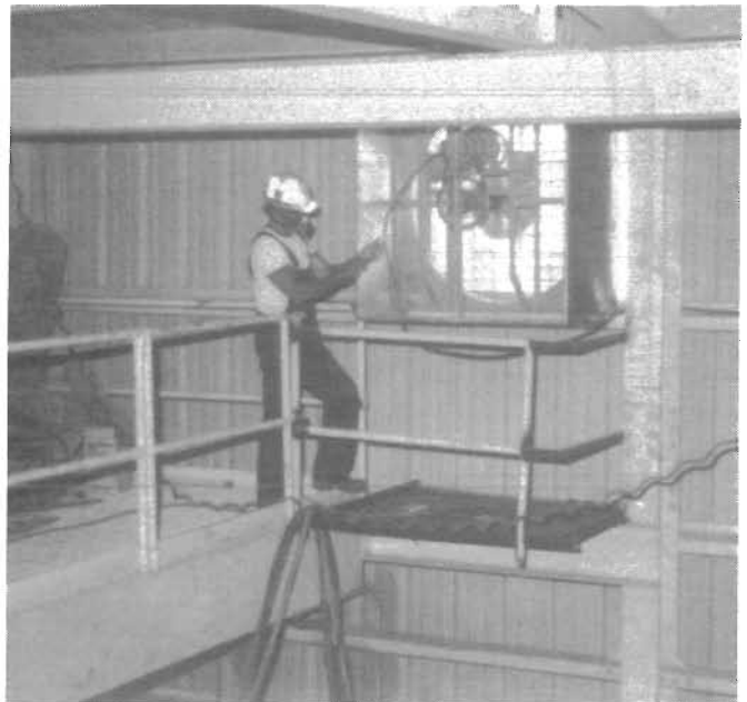
Figure 8.—Worker taking gas sample for tracer gas analysis at exhaust fan.
