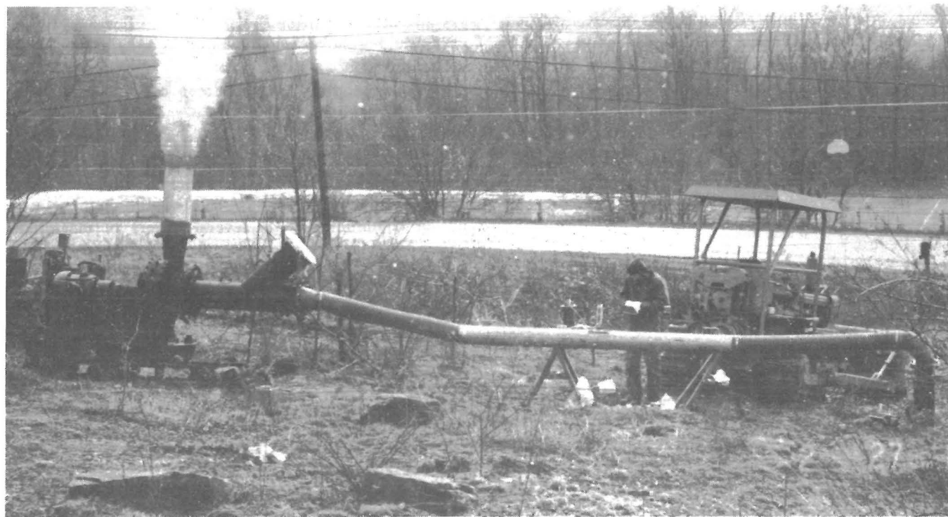
Figure 6.—Fan assembly in operation during borehole communications study.
