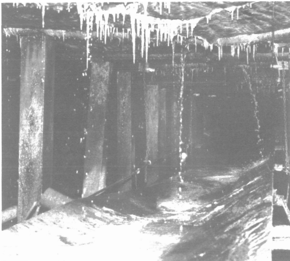
Figure 13.—Water inflows from mine roof.
