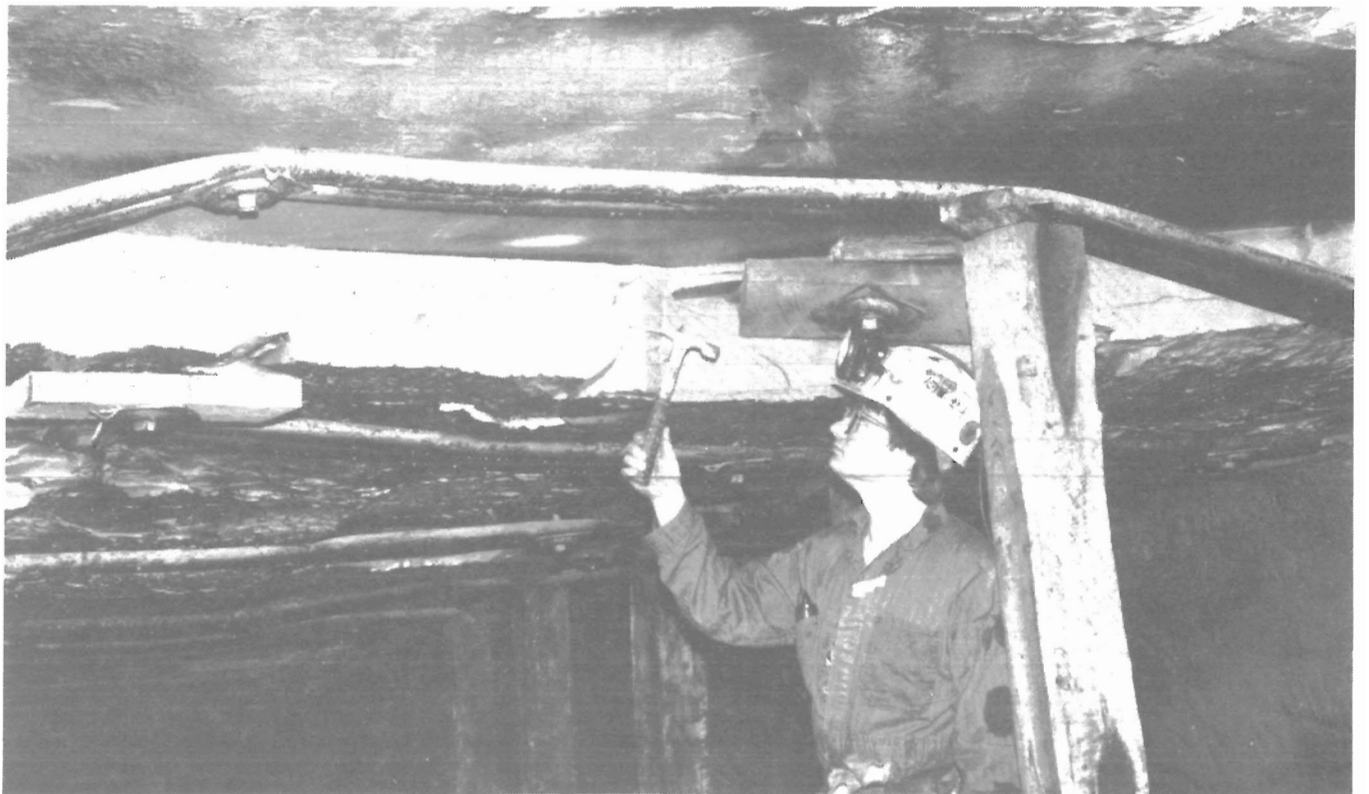
Figure 11.—Supplemental support of bad roof areas.
