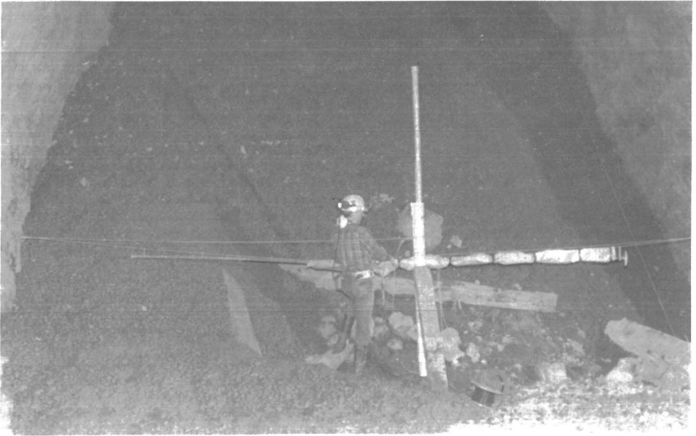
Figure 13.—Partially assembled horizontal and vertical backfill extensometers at toe of cemented backfill.
