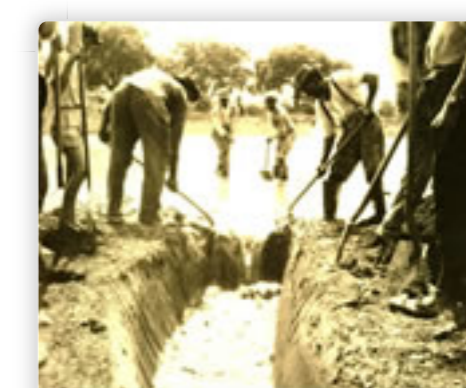
Drainage activities, Virginia, 1920's
