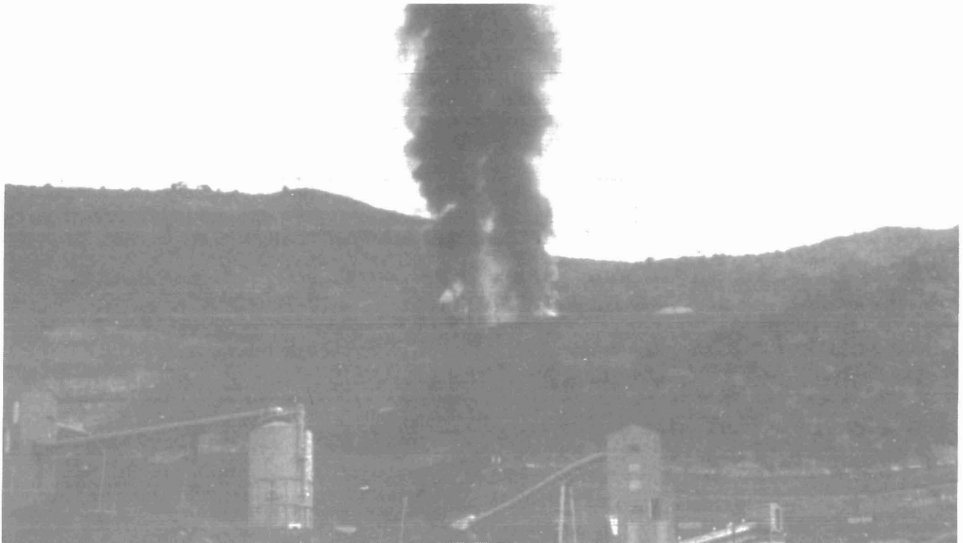
Figure 11.—Coal tars burning in fan and intake shafts.
