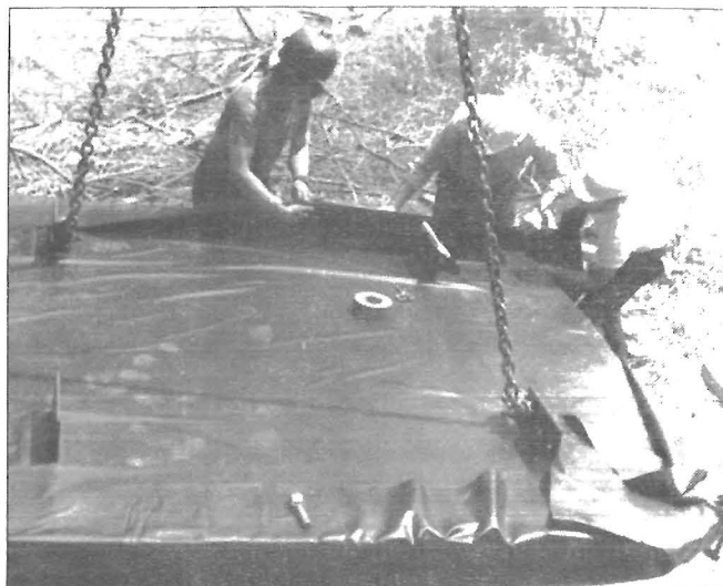
Figure 12.—Applying geomembrane covering to shaft platform.
