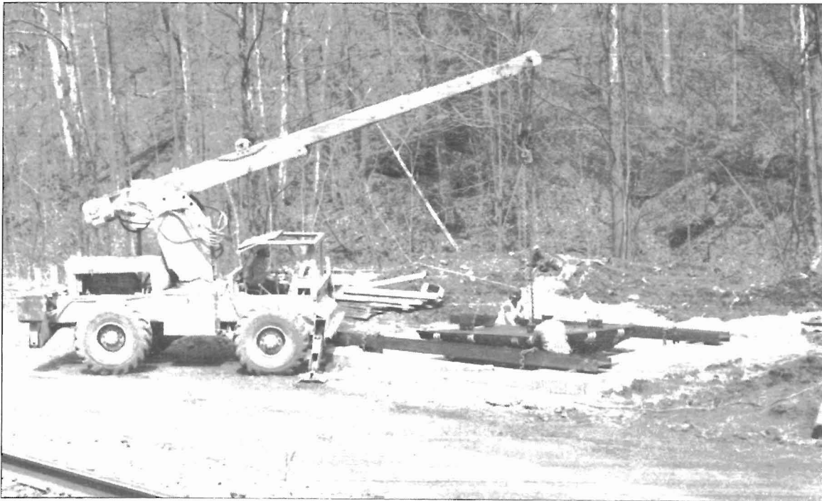
Figure 15.—Platform being lowered into shaft. Note beams in place alongside shaft.
