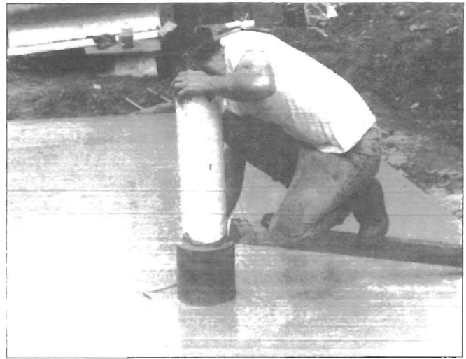
Figure 26.—Hand-packing grout between protective steel casing and vent tube.
