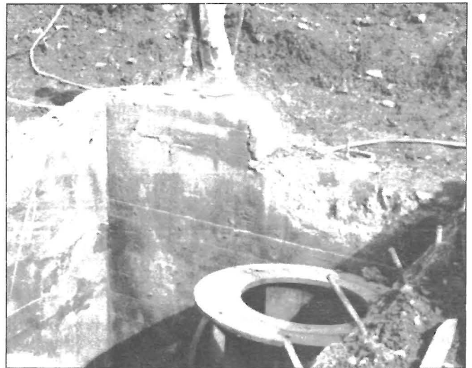
Figure 8.—Removing original concrete shaft collar with jackhammer.
