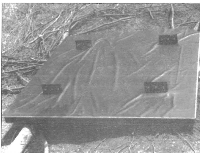
Figure 13.—Shaft platform wrapped with geomembrane.
