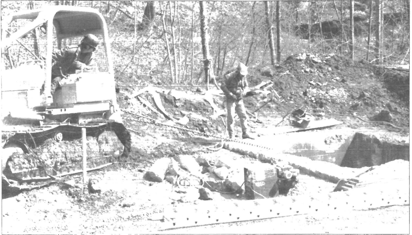
Figure 10.—Removing shaft utilities after removal of shaft collar.
