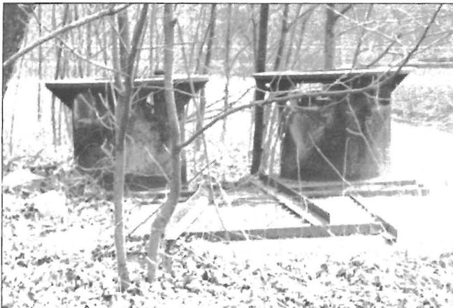
Figure 2.—Shaft site. Remnants of pump housing lie over abandoned shaft.
