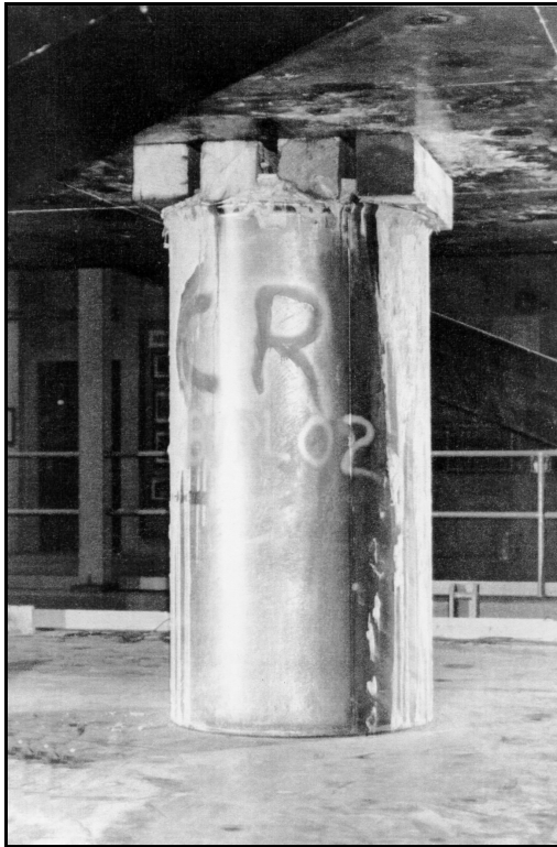
Figure 1.—Can crib used to replace wood crib in underground coal mines.
