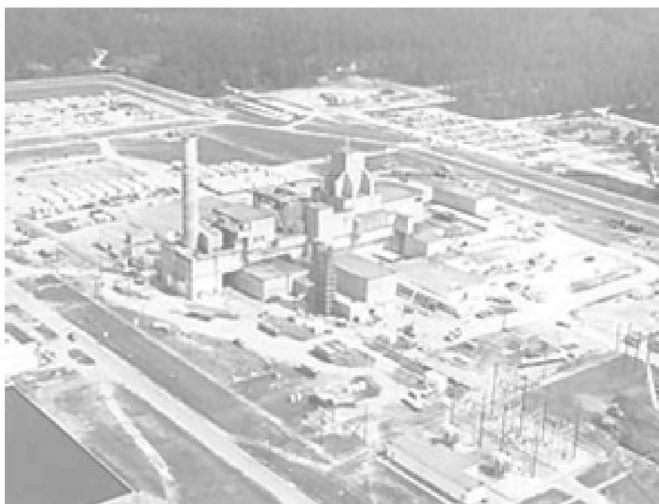
L-Reactor Facility. L Area, Savannah River Site, South Carolina. September 16, 1982. Photo courtesy of the U.S. Department of Energy.
