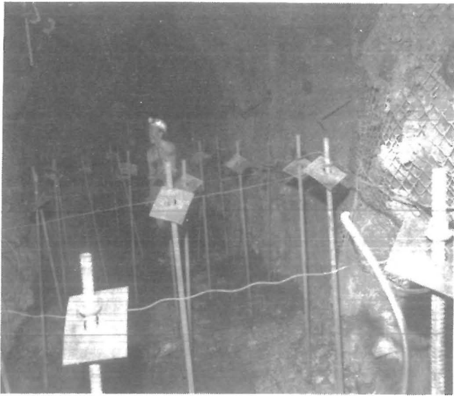
Figure 14.—Preparing Dywidag bolts for sandfill.
