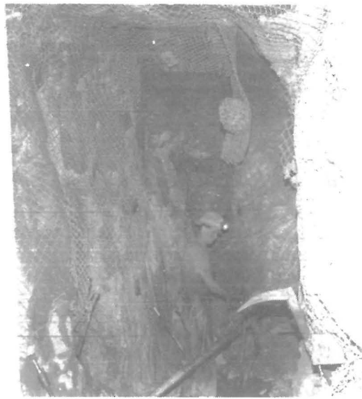
Figure 15.—Hanging chain link fencing for overhead protection.
